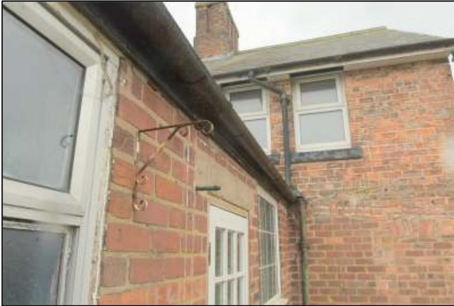
Gable is well sealed, no access to the wall top
