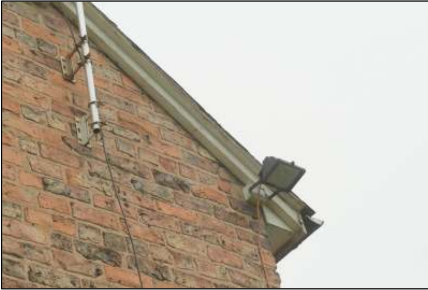
Timber soffits are all well sealed with no holes or cavities
