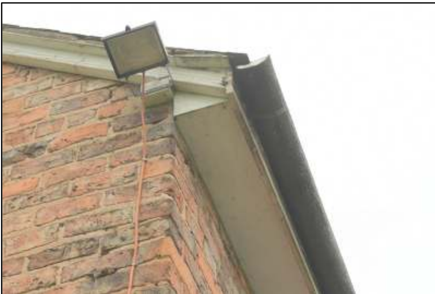
Timber soffits are all well sealed with no holes or cavities
