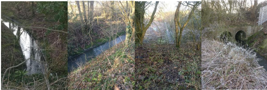
Figure 3 – Redwither Brook - Heavily Modified Channel and Culvert
