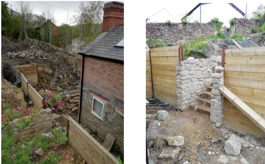
Fig. 3&4 – Pictures of partly constructed retaining wall
