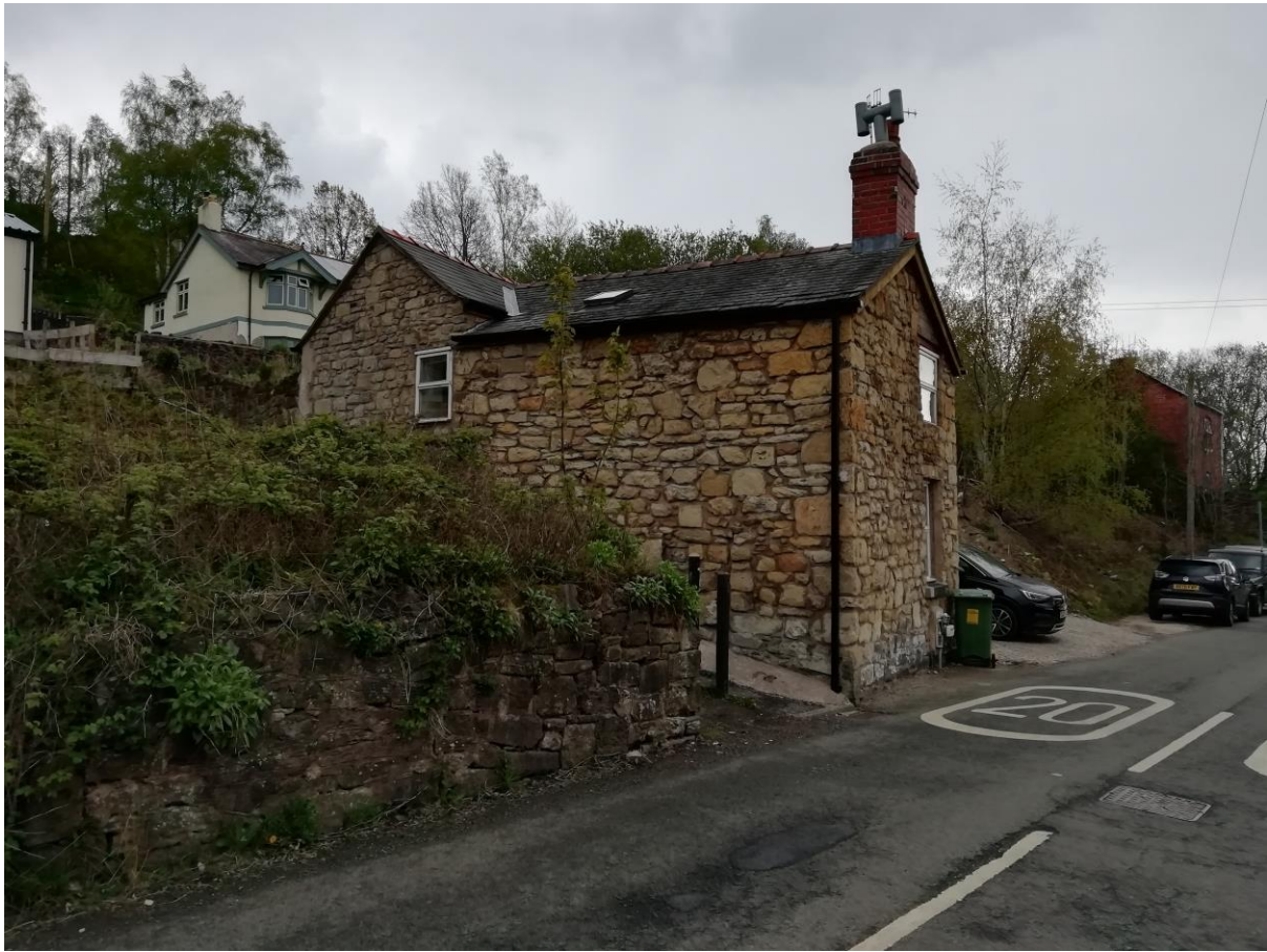
Fig. 2 – Picture of Existing North Elevation
