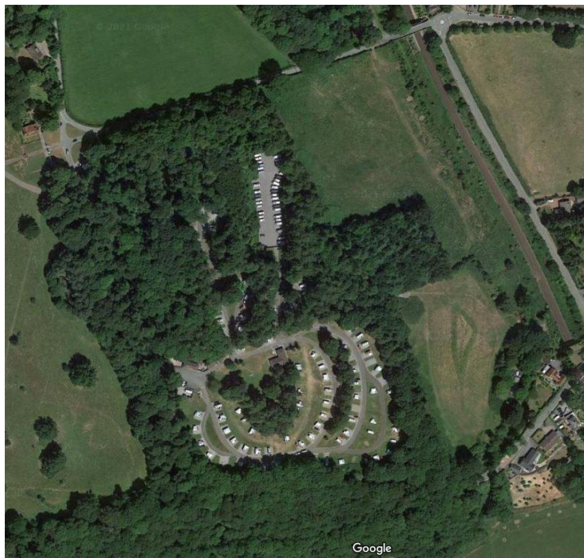
Aerial view of site
