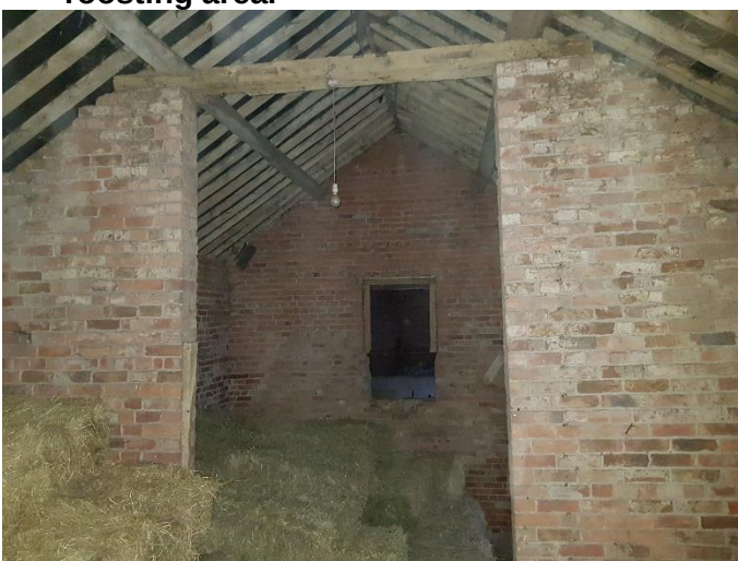
Hay barn extending into north wing of the barn range. This area was in use by Brandt's bats for foraging and will remain undeveloped but will house the compensatory roost sites.
