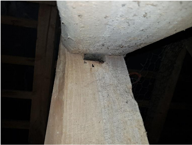
One of the suspected roosting sites for soprano pipistrelle within the loft above the west wing.
