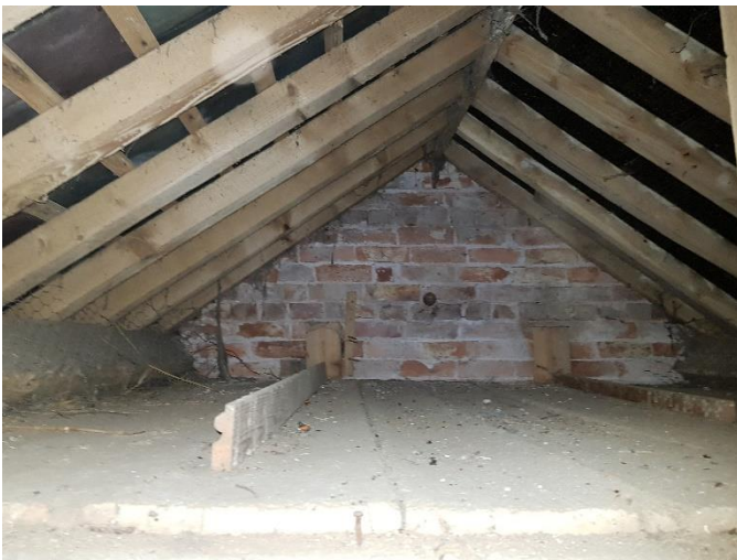
Enclosed area within loft space above the west wing. Suspected common pipistrelle night time roosting area.
