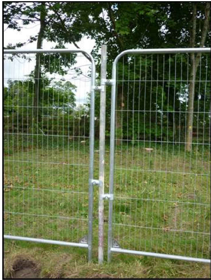
Tree Protective Fencing Specification
