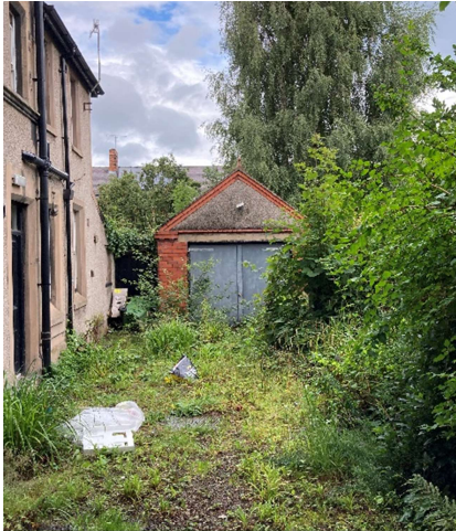
(Fig 5) Existing garage building
