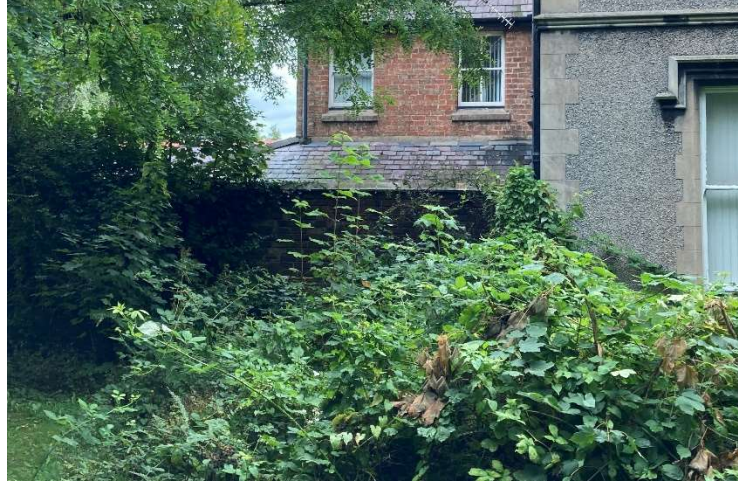
(Fig 6) Existing garden wall, screened in foliage.
