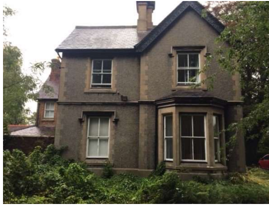
(Fig 3) Existing south west gable
