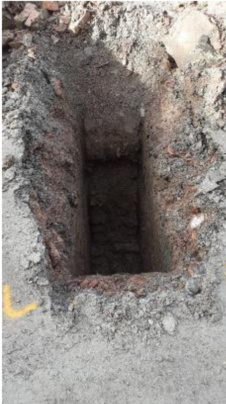
PLATE 3 VIEW OF TP108 EXCAVATION
