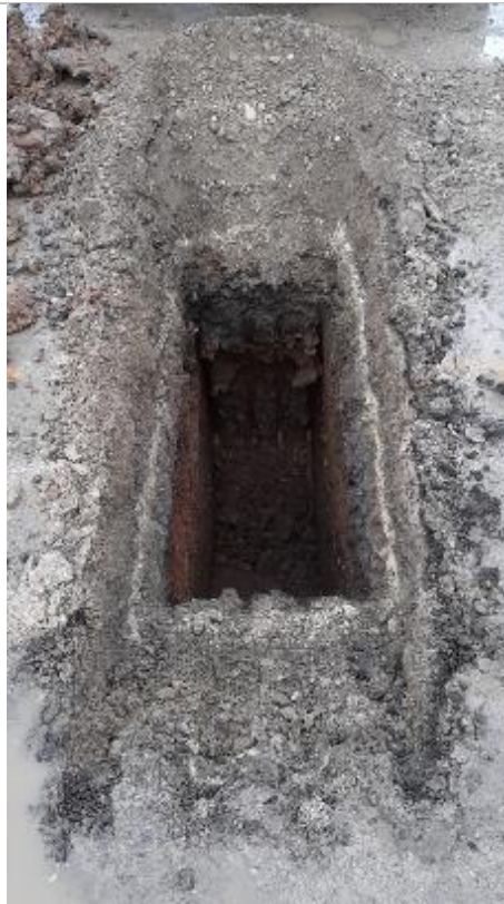
PLATE 4 VIEW OF TP110 EXCAVATION
