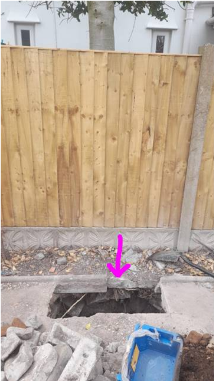
Minor feeder roots just below the concrete bound surface
