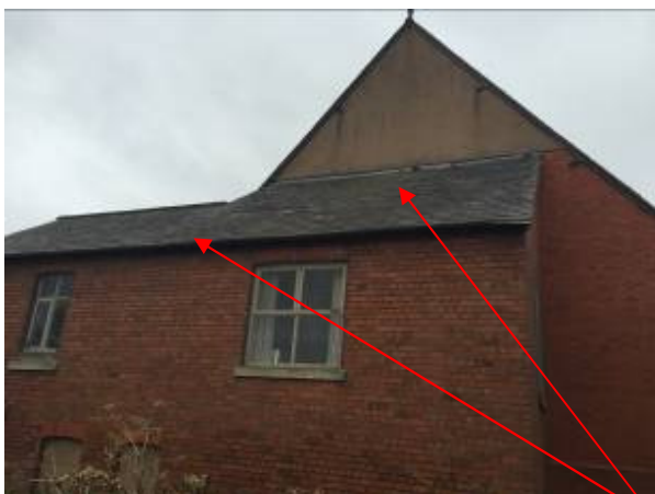
Gaps at lead flashing, under eaves and between fascia boards & external brickwork
