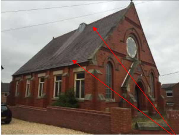
Salem Chapel proposed for demolition – gaps under roof slates
