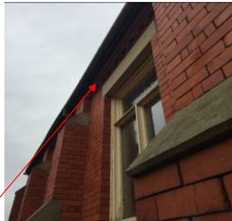
Gaps at lead flashing, under eaves and between fascia boards & external brickwork
