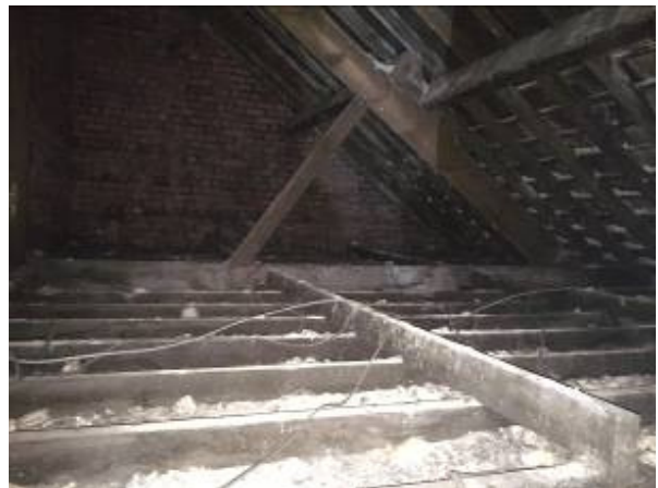
Loft space above church hall to the north
