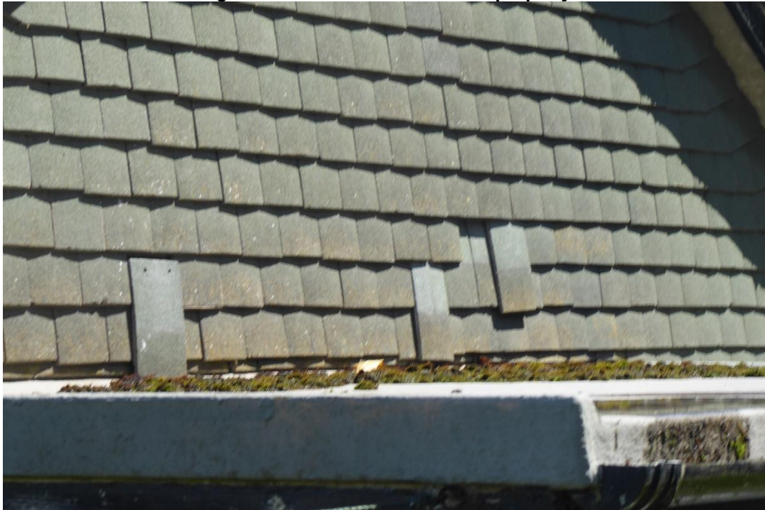
Figure 5. Hanging tiles on southwest gable
