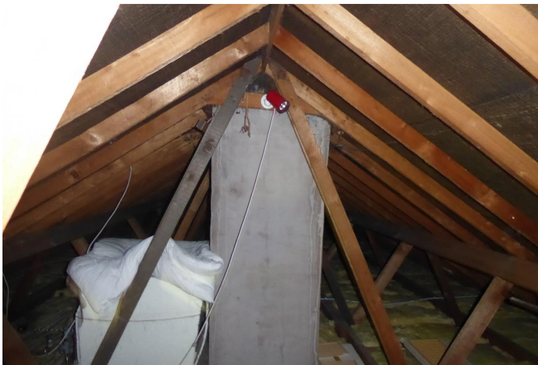
Figure 6. Interior of roof void
