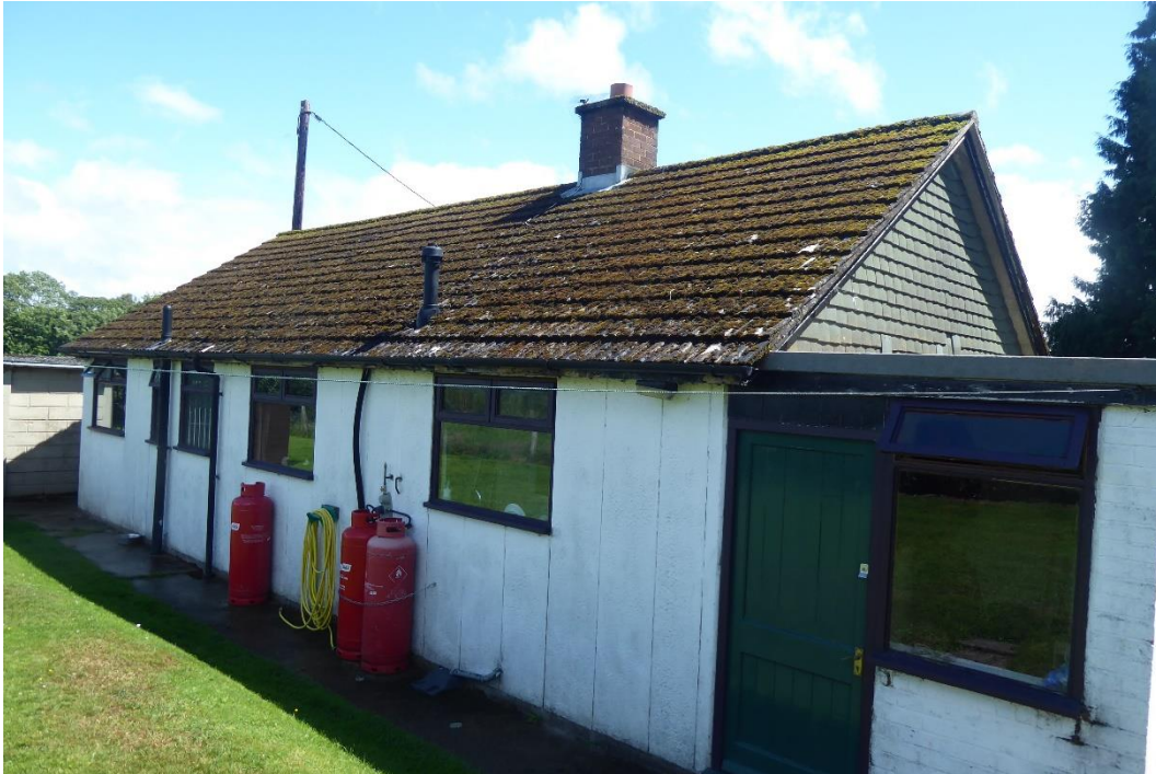
Figure 4. Southwest elevation of property
