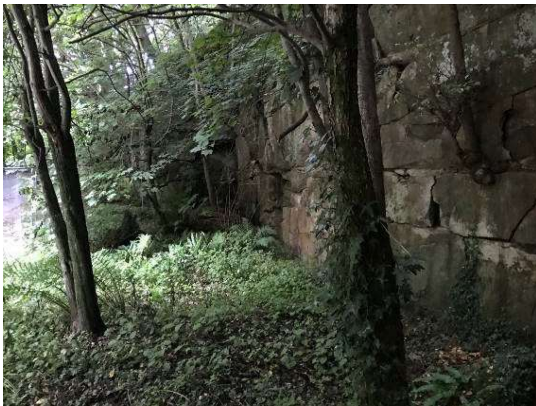
Photo 4 – 19m long rock face, offset by c. 7m from verge
