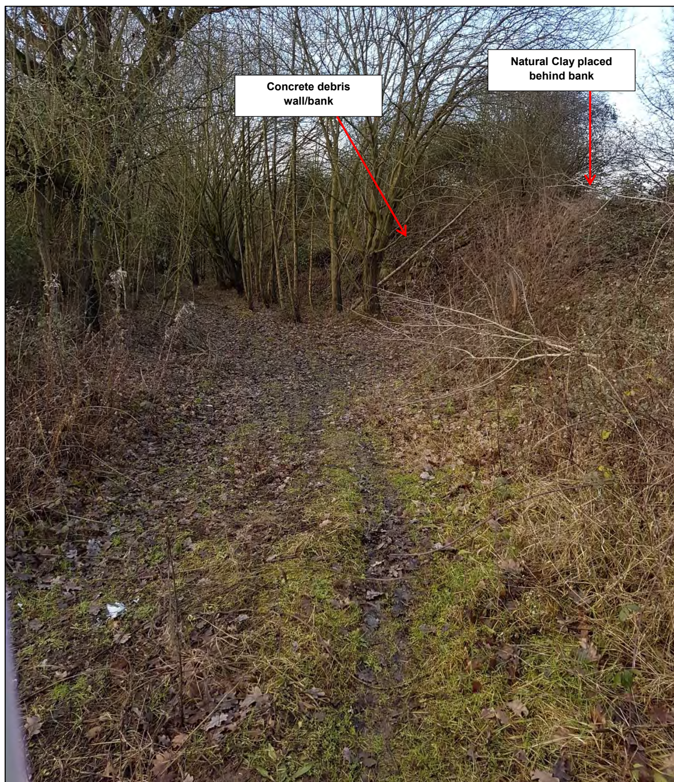
Photograph 18: SW of the proposed development area. Photo showing extent of concrete debris wall/bank created from magazine buildings demolition material
