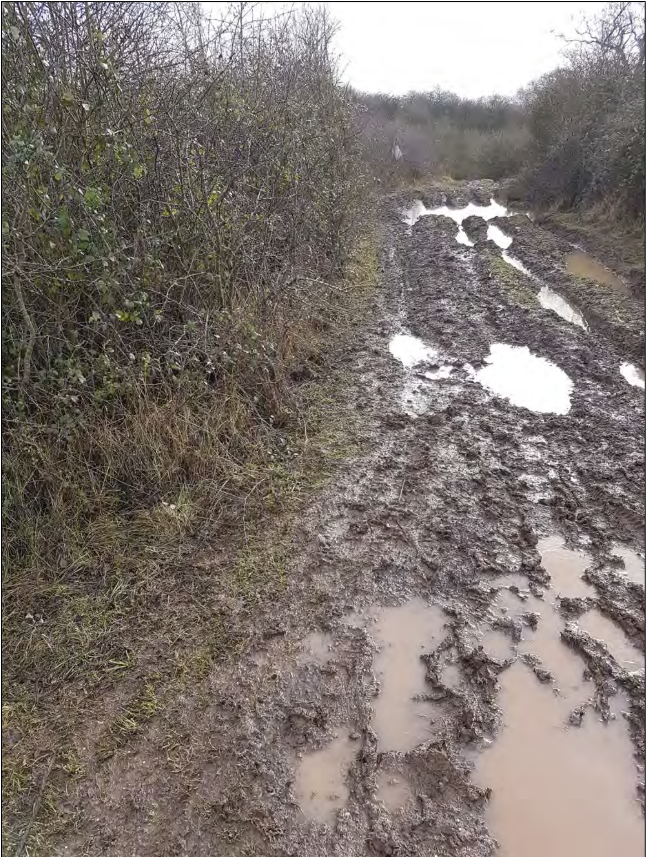
Photograph 17: North eastern area of the proposed development.
