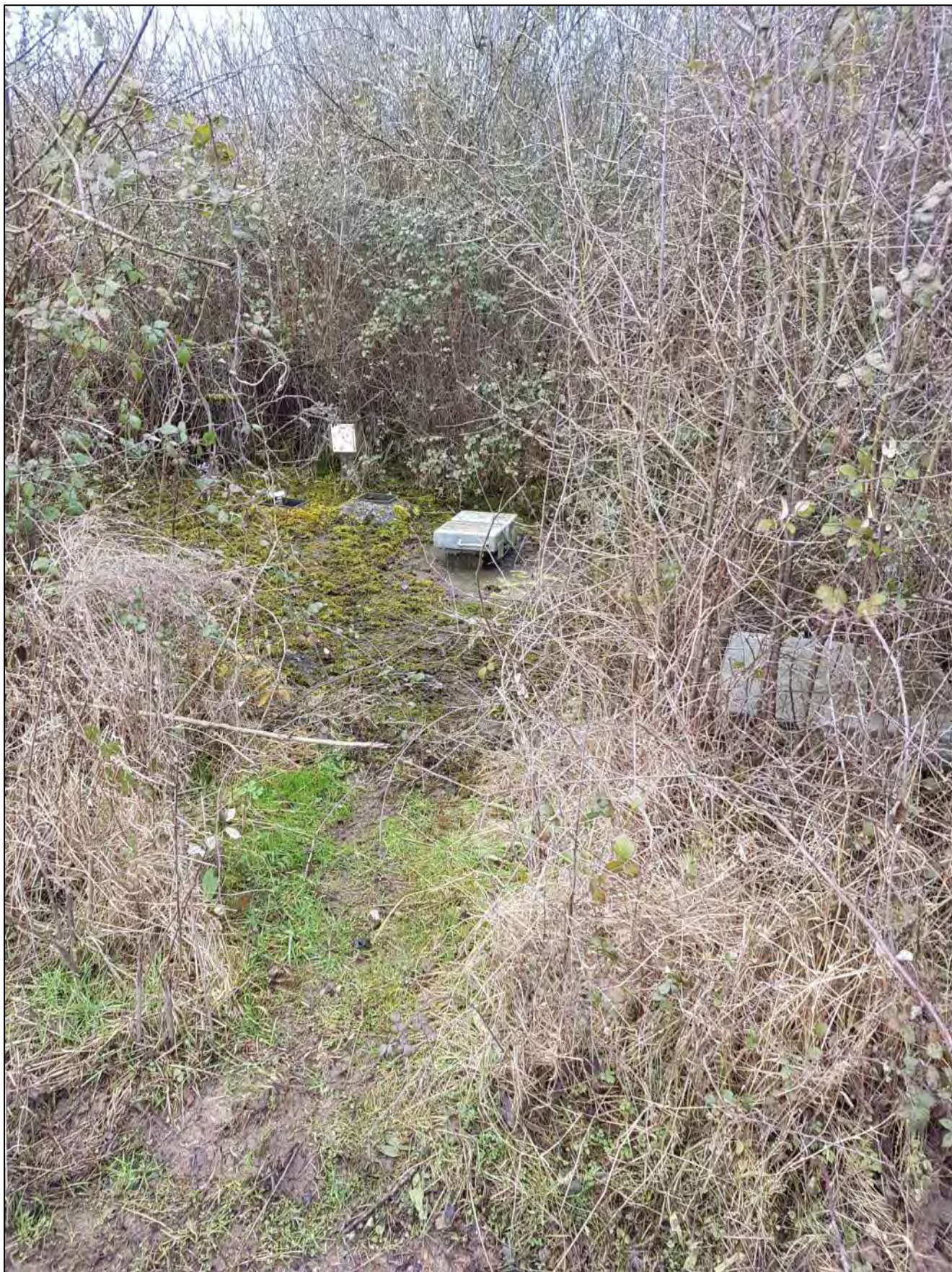
Photograph 3: Chambers for waters services noted to run parallel with part of the eastern access track.
