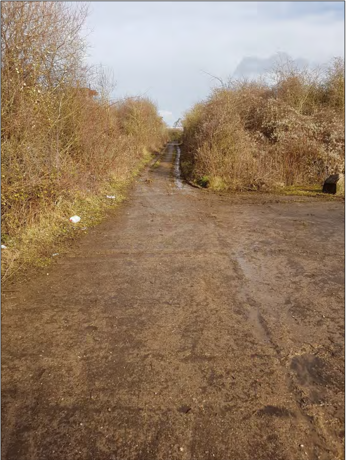
Photograph 1: Looking north east along the eastern access track.
