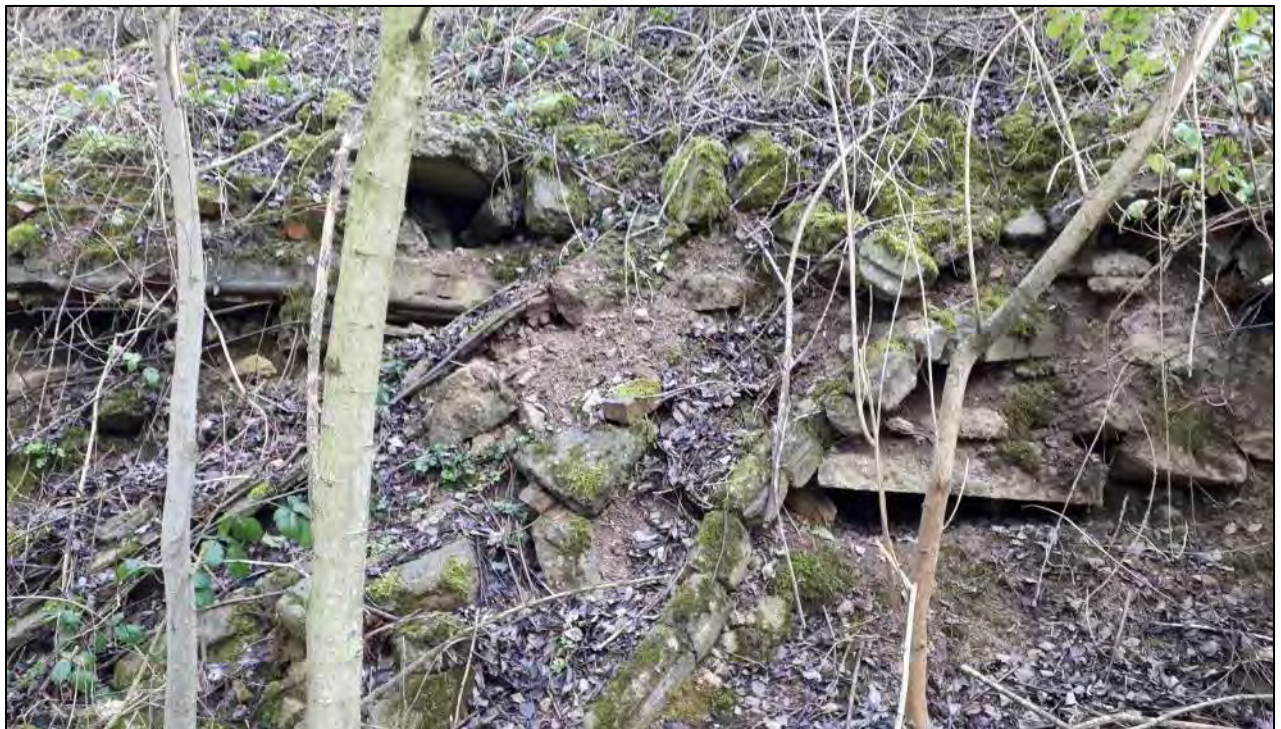
Figure 8: Photo from SW boundary showing wall made from concrete material of the demolished magazine buildings. Natural Glacial Clay from Kellogg's was placed behind.
