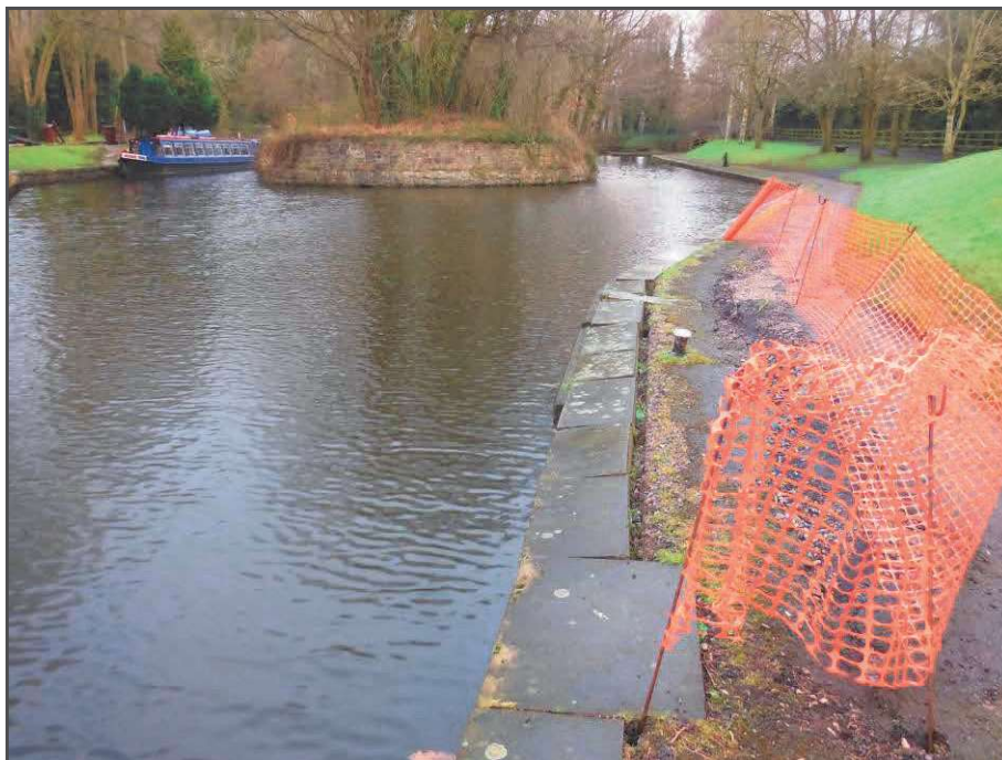
Photograph 5: View north-east towards the eastern canal arm and wharf.
