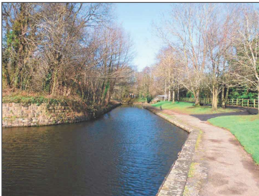
Photograph 6: View north-east along the eastern canal arm and wharf.
