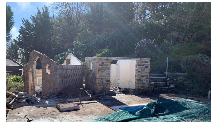
Image of Previous Pool Structures
