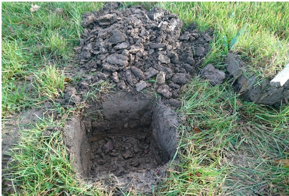
Figure 3-5: Trial Pit in Field 1C – terminated due to low observed rates of infiltration
