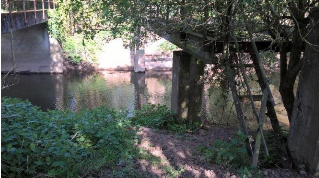
Figure 3-11: Bridge structures at downstream end of Site (CLYW1615)
