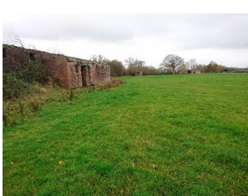
(a) South-west towards existing solar farm
