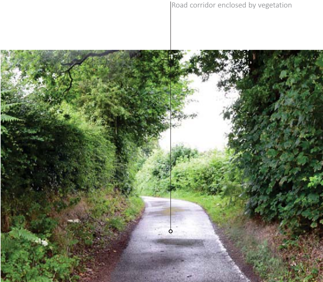
Photo 4.1 - View from Sandy Lane looking north.
