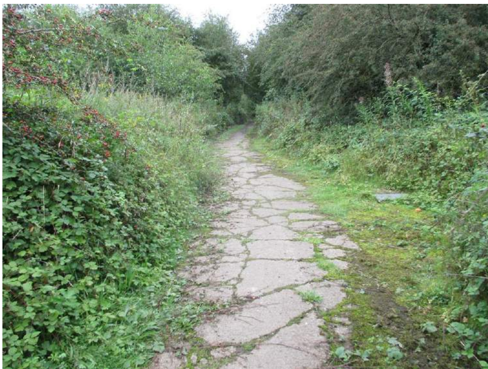
Plate 8: Typical view along the concrete paths on the site.
