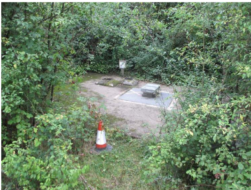
Plate 15: View of the water chamber covers located in the north east area of the site looking north west.
