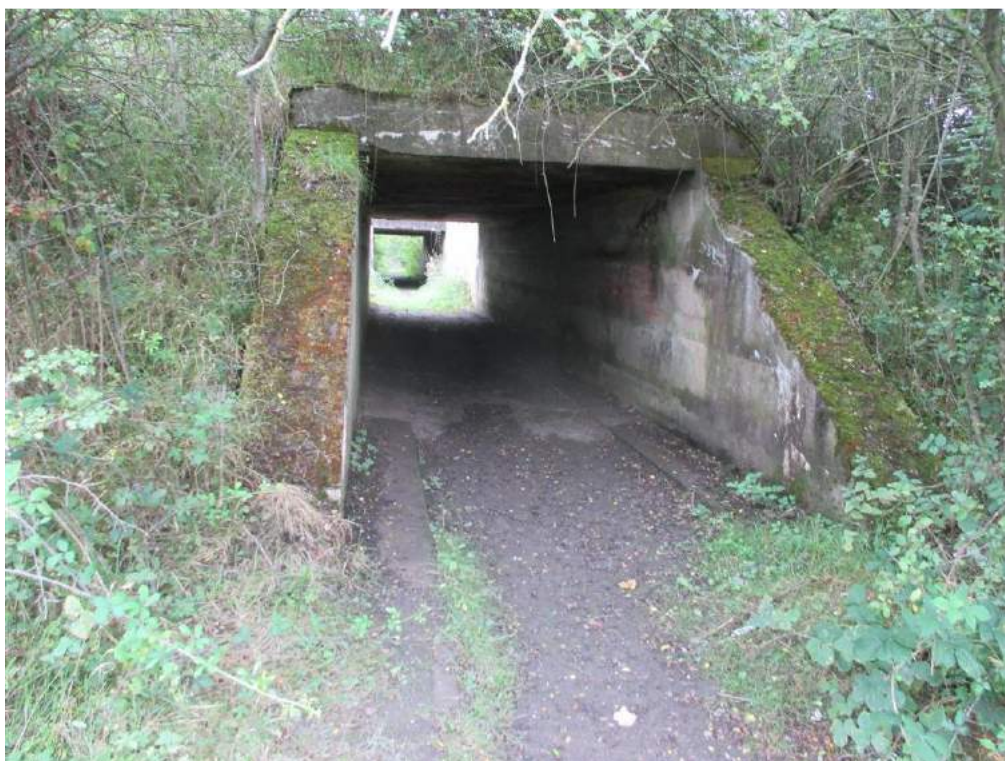
Plate 11: Typical example of concrete box tunnels on site.
