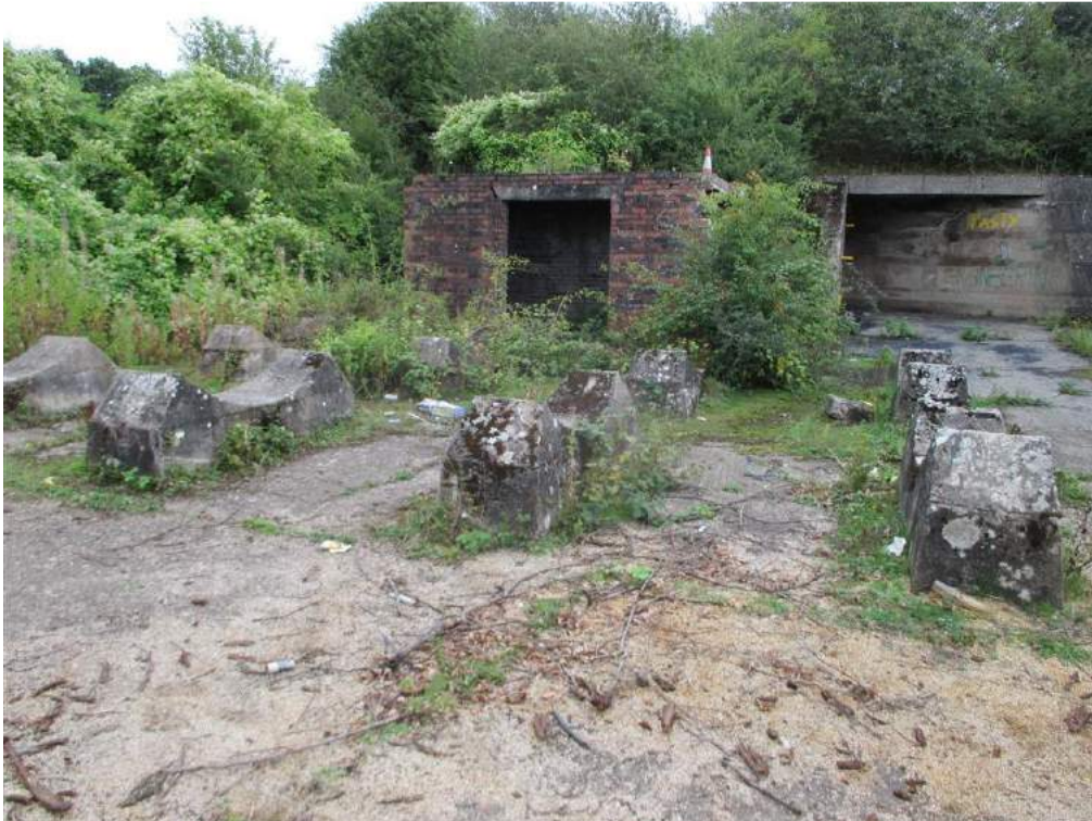
Plate 13: Tank cradles located in the north east area of the site.
