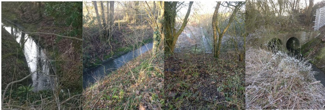
Figure 3 – Redwither Brook - Heavily Modified Channel and Culvert
