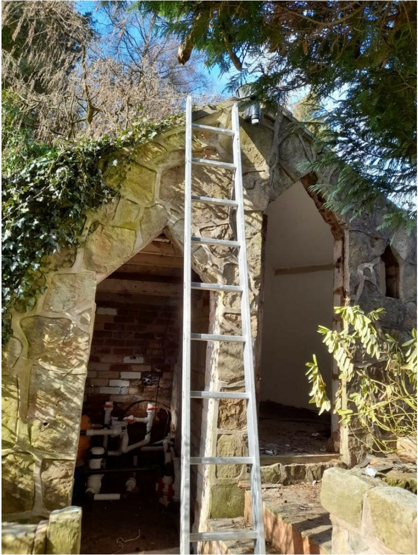
PHOTO 2- Existing Pump House
