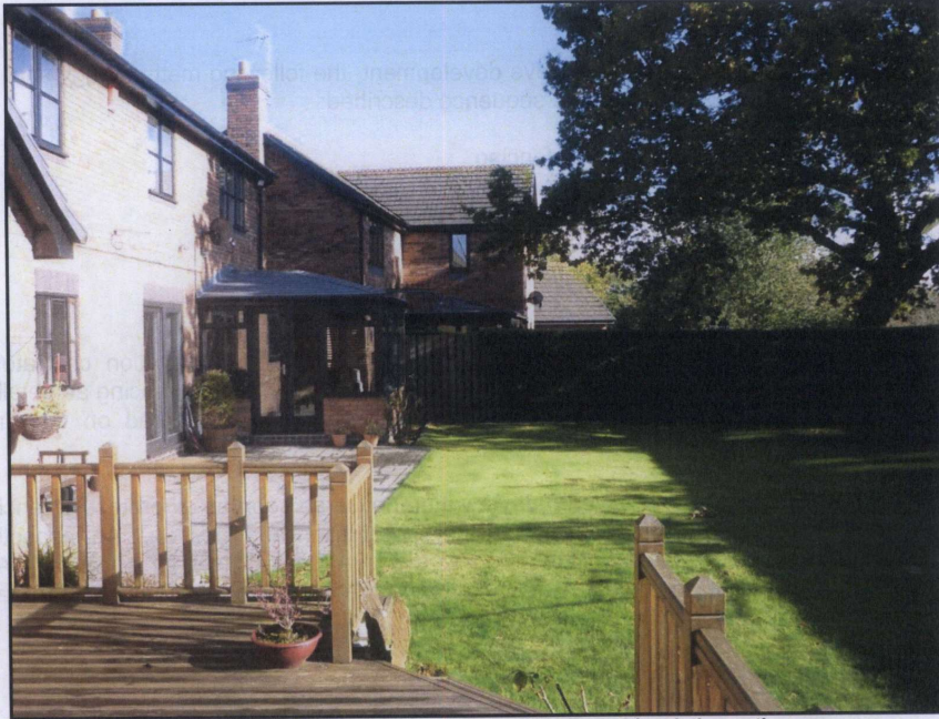
Photo 1 - Location of extension approximately in line with existing patio area
