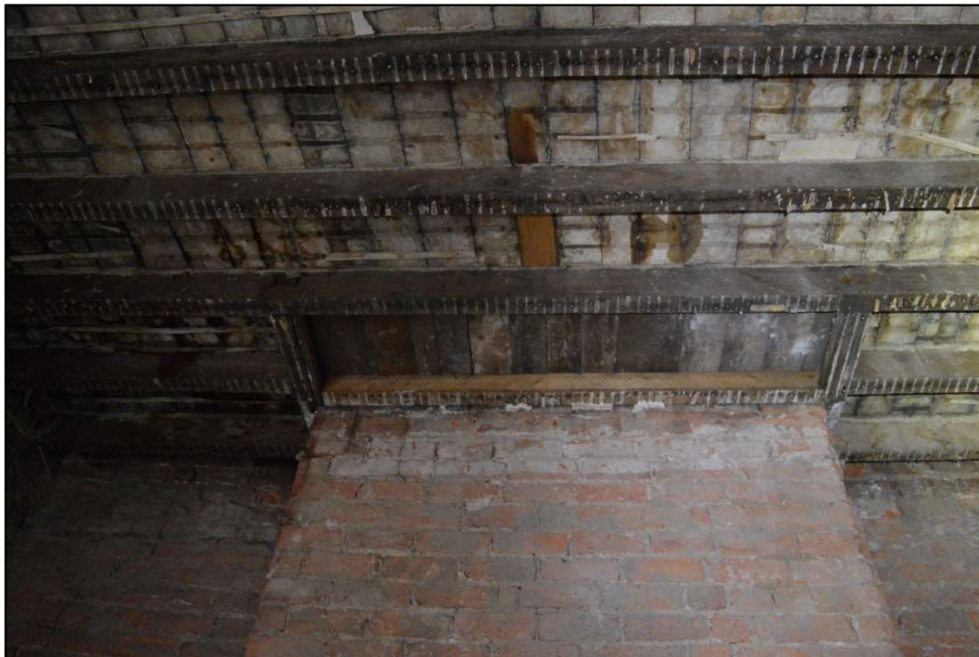
Fig 32: As 31. Top of chimney breast in Room 8 on first floor showing supporting timber for the hearth stone (CPAT 4853-0031)
