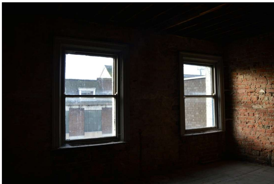
Fig 11: Windows in Room 3 on second floor (CPAT 4853-0010)
