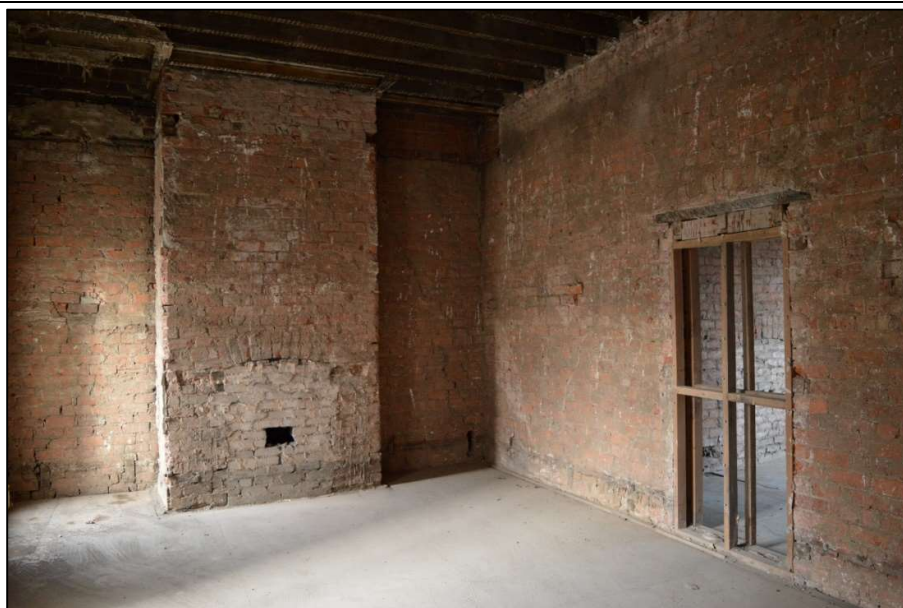
Fig 39: Blocked fireplace and door in Room 6 on first floor. Also shows wall cracks (CPAT 4853-0038)
