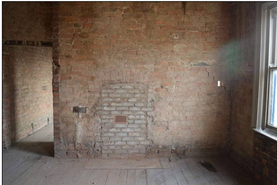
Fig 12: Blocked fireplace with hearth stone in Room 3 on second floor. Also shows wall cracks (CPAT 4853-0011)
