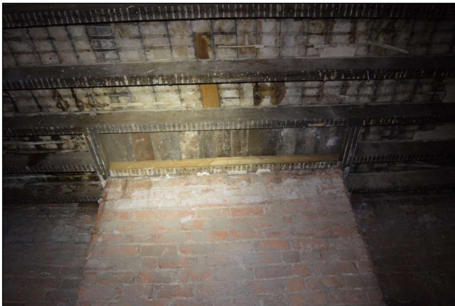
Fig 31: Top of chimney breast in Room 8 on first floor showing supporting timber for the hearth stone (CPAT 4853-0030)
