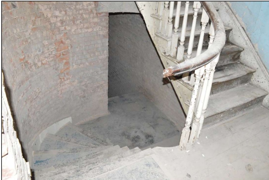
Fig 68: Looking down the east stair from the first floor landing. Shows where the east stair was truncated by the modern insertion of steps down (centre) to the rear of the building (CPAT 4853-0066)
