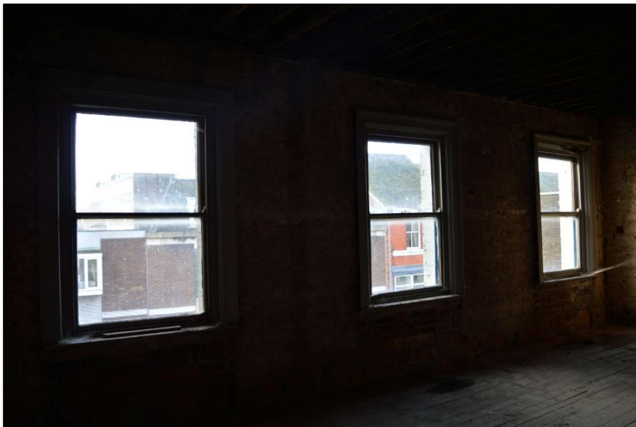
Fig 7: Windows in Room 2 on second floor (CPAT 4853-0006)
