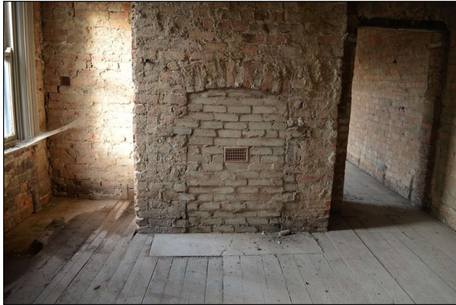
Fig 10: Blocked fireplace with hearth stone in Room 2 on second floor. Also shows wall cracks (CPAT 4853-0009)
