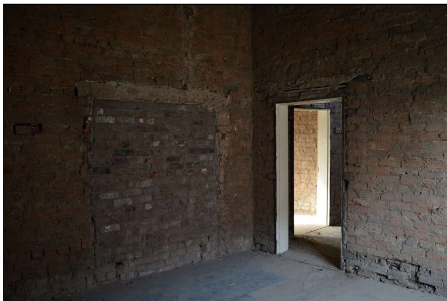
Fig 29: Blocked doorway in Room 8 on first floor. Also shows doorway to west stair (CPAT 4853-0028)
