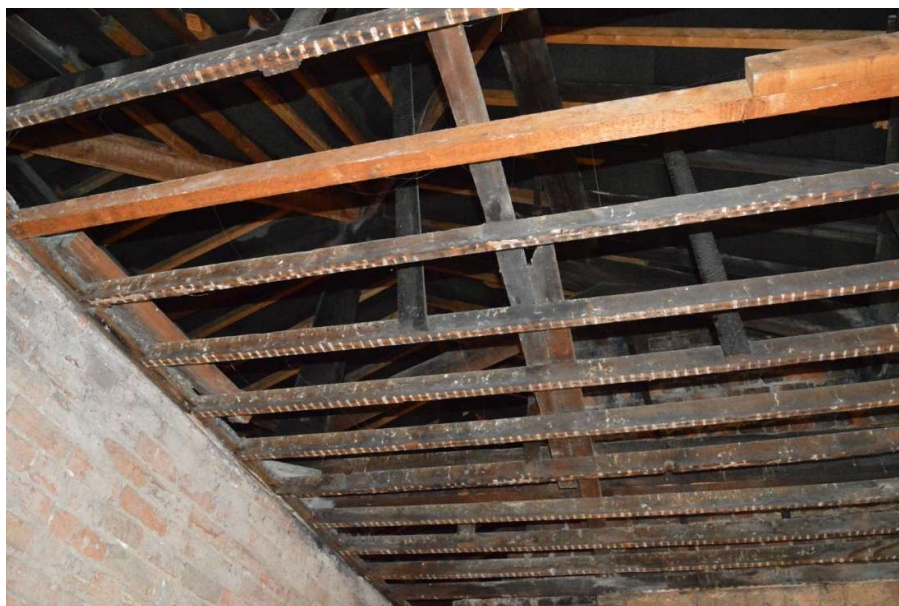
Fig 70: Ceiling timbers with Truss 4 behind in roof space (CPAT 4853-0069)
