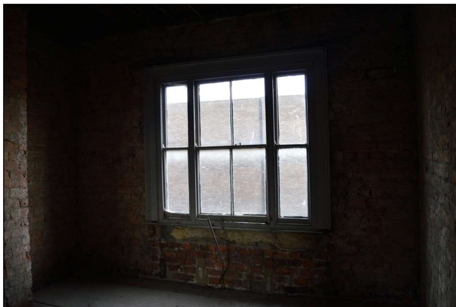
Fig 5: Window in Room 1 on second floor (CPAT 4853-0004)
