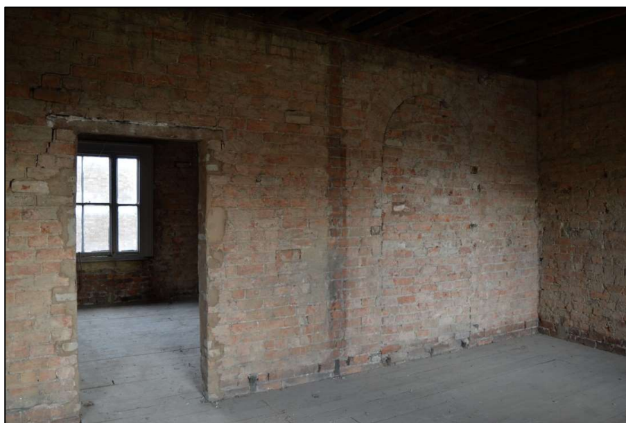
Fig 9: Blocked arched doorway and ?later doorway in Room 2 on second floor (CPAT 4853-0008)
