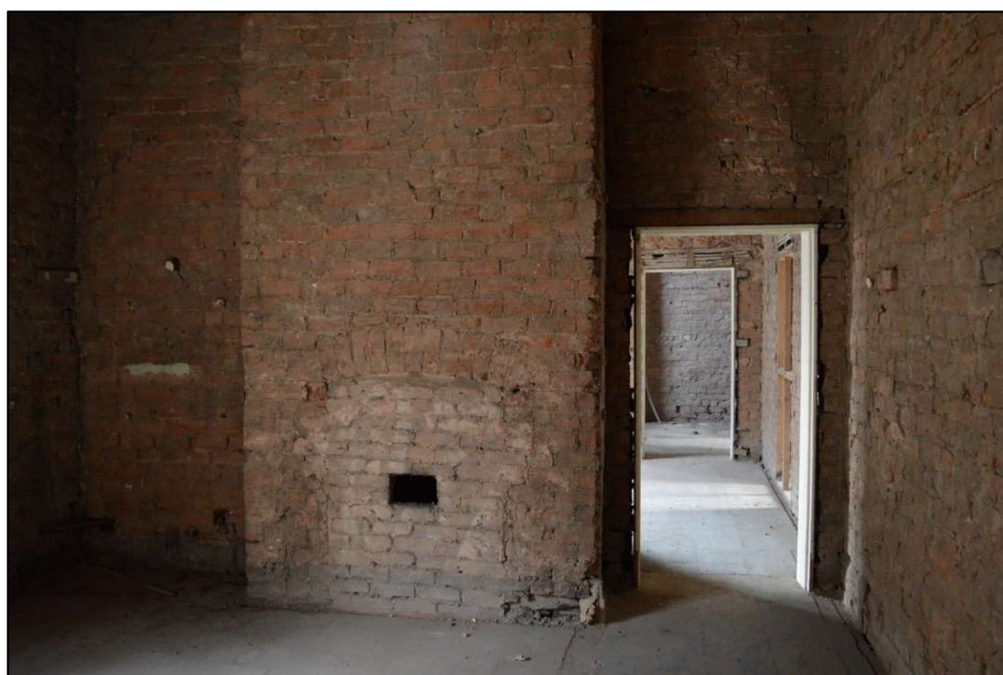
Fig 27: Blocked fireplace in Room 8 on first floor and route to east stair (CPAT 4853-0026)
