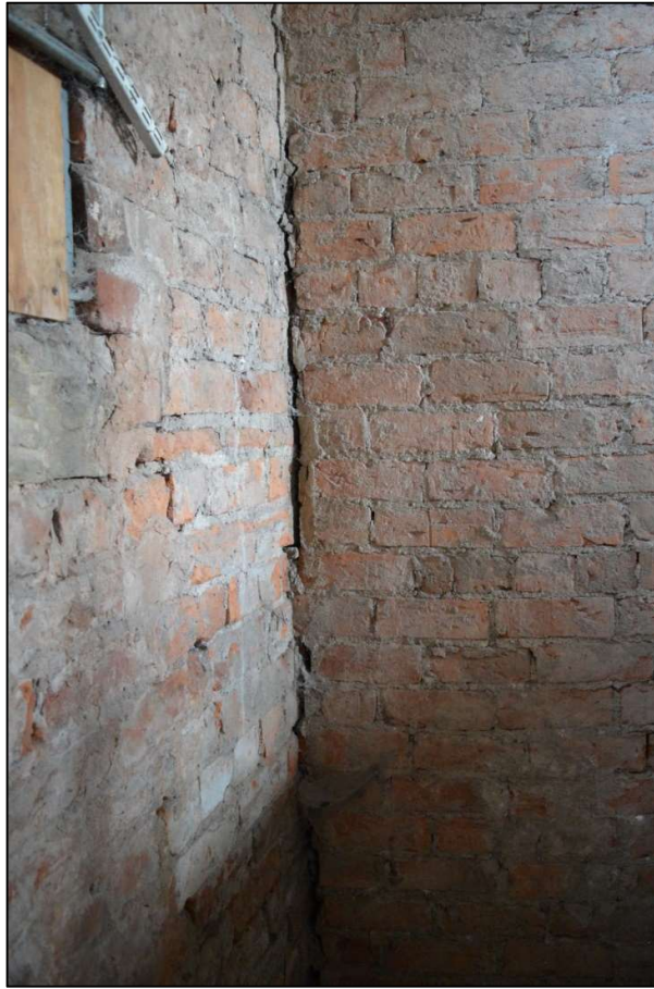
Fig 20: Poorly tied-in and possibly inserted wall (to right) on east side of west stair (CPAT 4853-0019)
