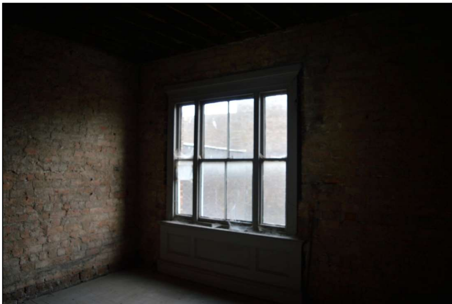
Fig 15: Window in Room 4 on second floor (CPAT 4853-0014)
