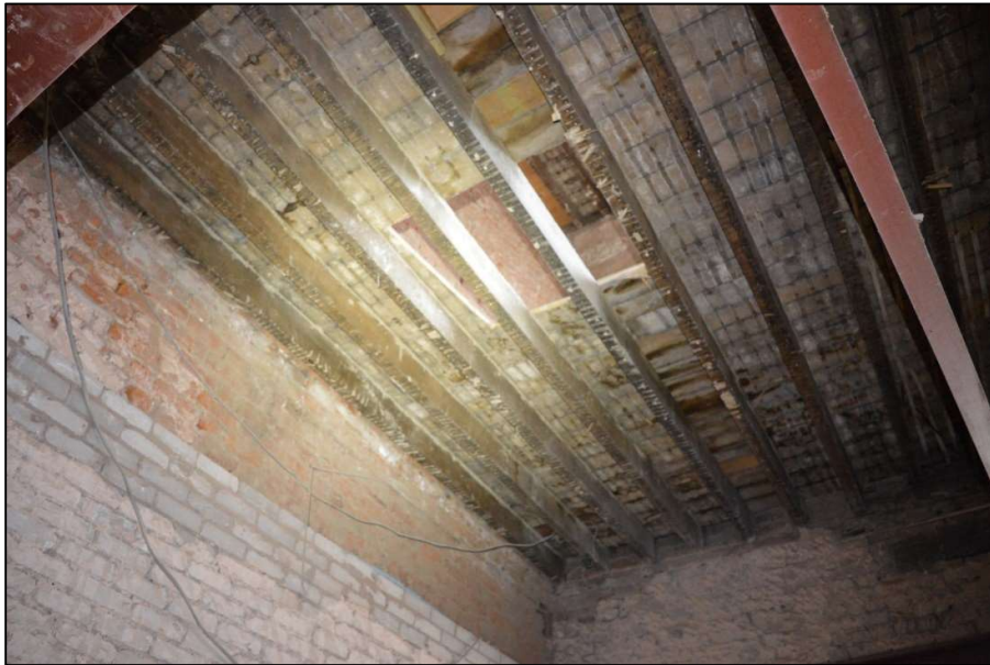
Fig 48: First floor supporting joists from below. Also shows original east wall (to left) of ground floor with modern brick facing of its lower part and the surviving upper part of the south wall (to right) of the original building (CPAT 4853-0047)
