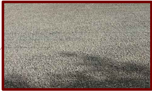
New Road and Parking Materiality – Permeable Hard Standing
