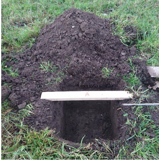
Pit A (dry)
