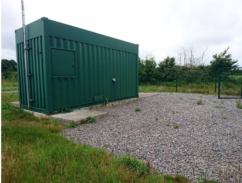
Figure 2-13: Typical layout showing gravel chippings around infrastructure on concrete pads
