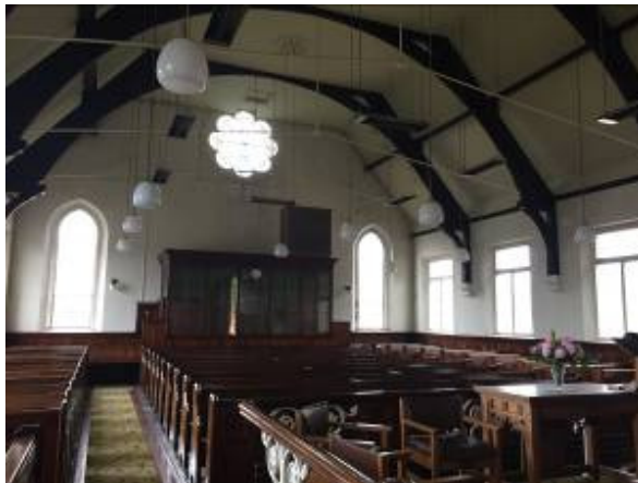
Light filled interior of chapel
