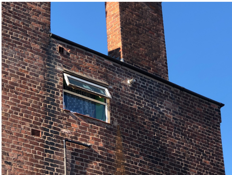
FIGURE 1: Image of the rear elevation where flue to be positioned.
