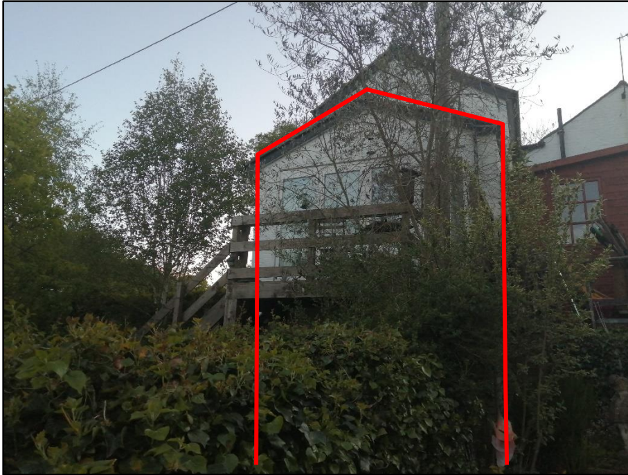
A1.1 Plate 1: View of the extension to be replaced
