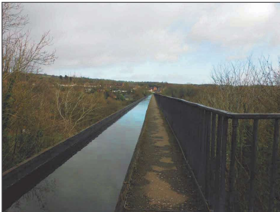
Photograph 43: View north-east along the Pontcysyllte Aqueduct (NMR 34410).
