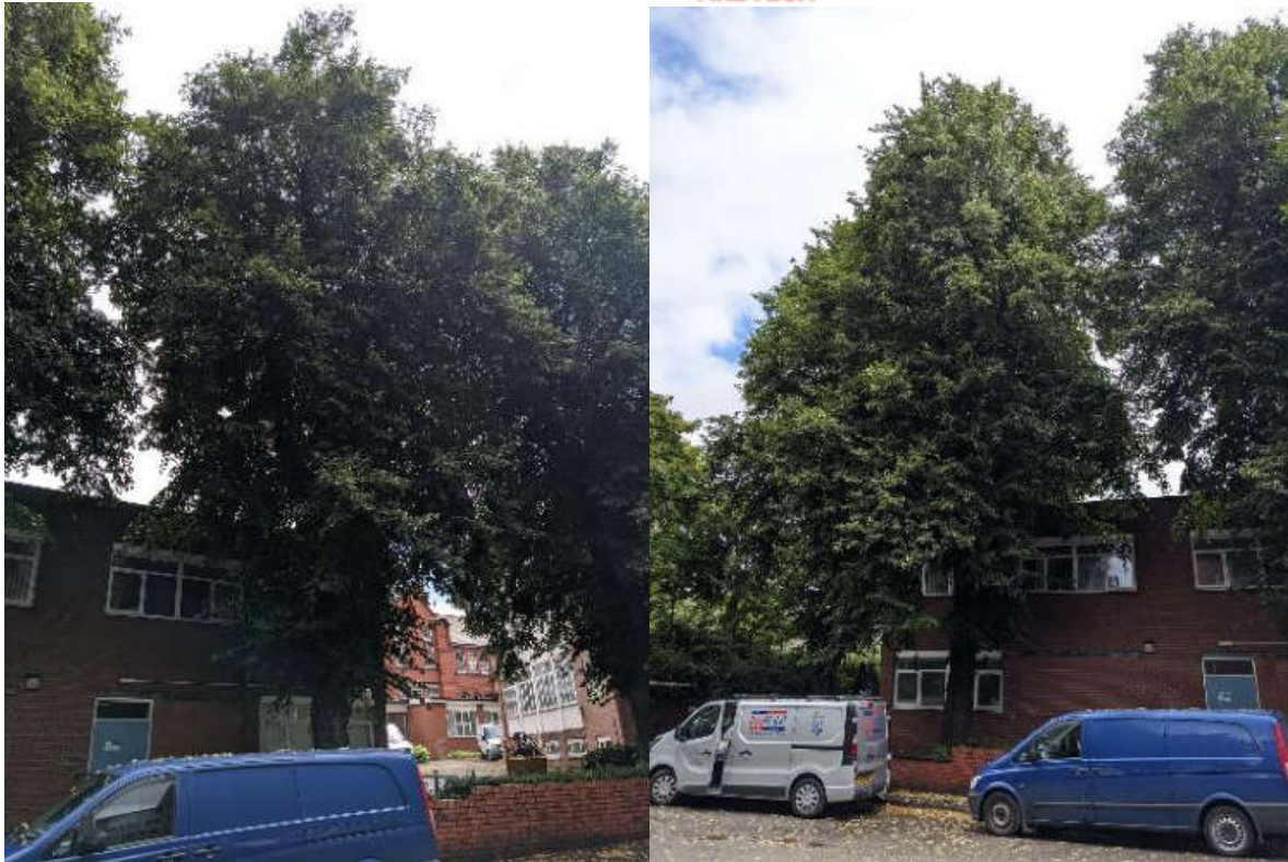
Figure 19. Tree 13 (left) and tree 14 (right) showing crown proximity to the adjacent building (both common limes).
