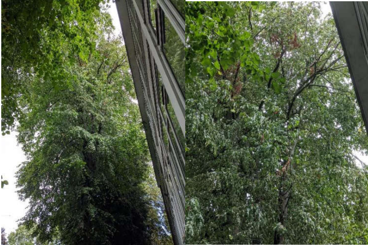
Figure 25. Tree 18 (common lime) crown proximity to adjacent building.
