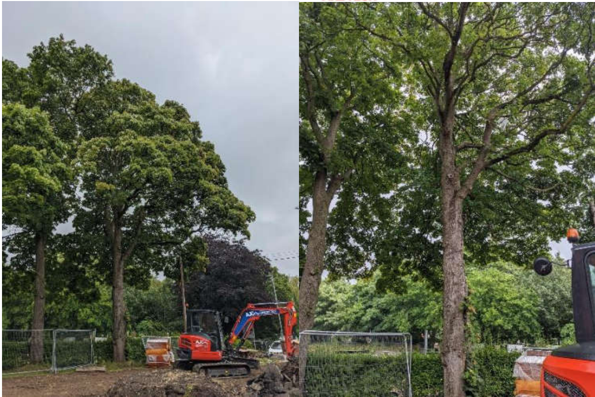
Figure 43. Trees 31, 32, and 33(sugar maples) and their proximity to the current construction work.
