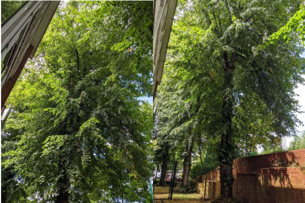
Figure 23. Tree 16 (common lime) crown proximity to adjacent building.
