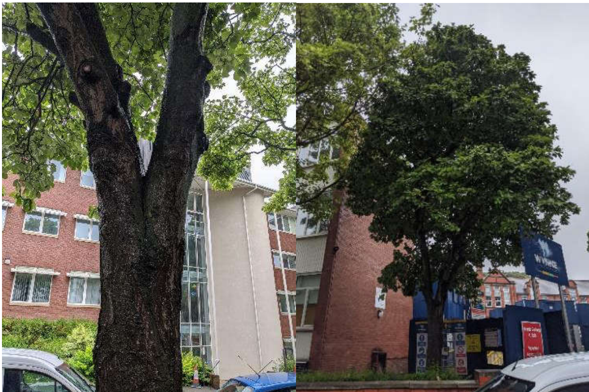
Figure 14. Tree 7 (Swedish whitebeam)) with slight bark inclusion and proximity to building.
