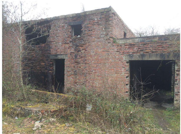
24- Exterior of Building 8
