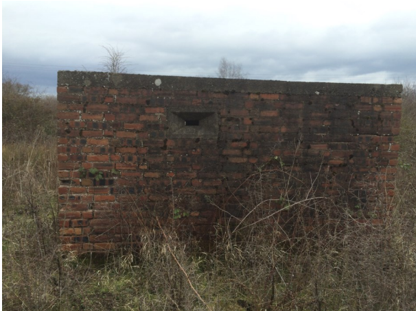
25- Typical pill box at site (B7)
