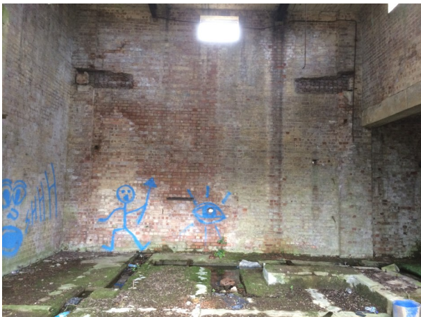
23- Interior of Building 3
