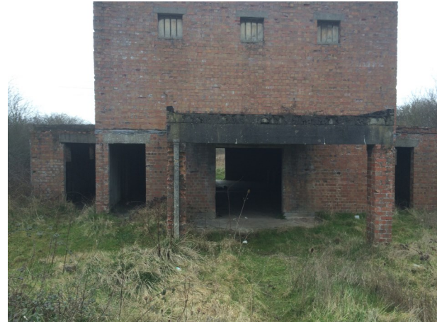
28- Exterior of Building 1
