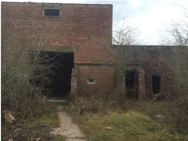
27- Exterior of Building 3
