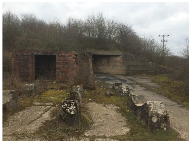
30- Exterior of Building 5 showing tunnel
