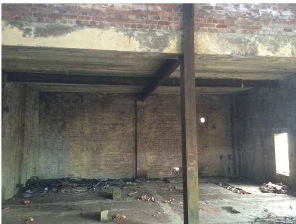
29- Interior of Building 3
