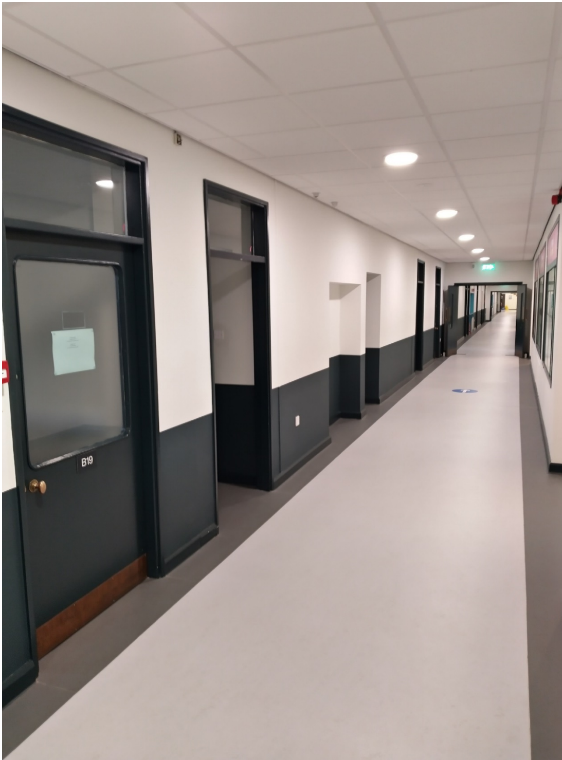
Image EDP 3: View along the central corridor in Block B illustrating preserved original door and recesses in respect of former entrances.
