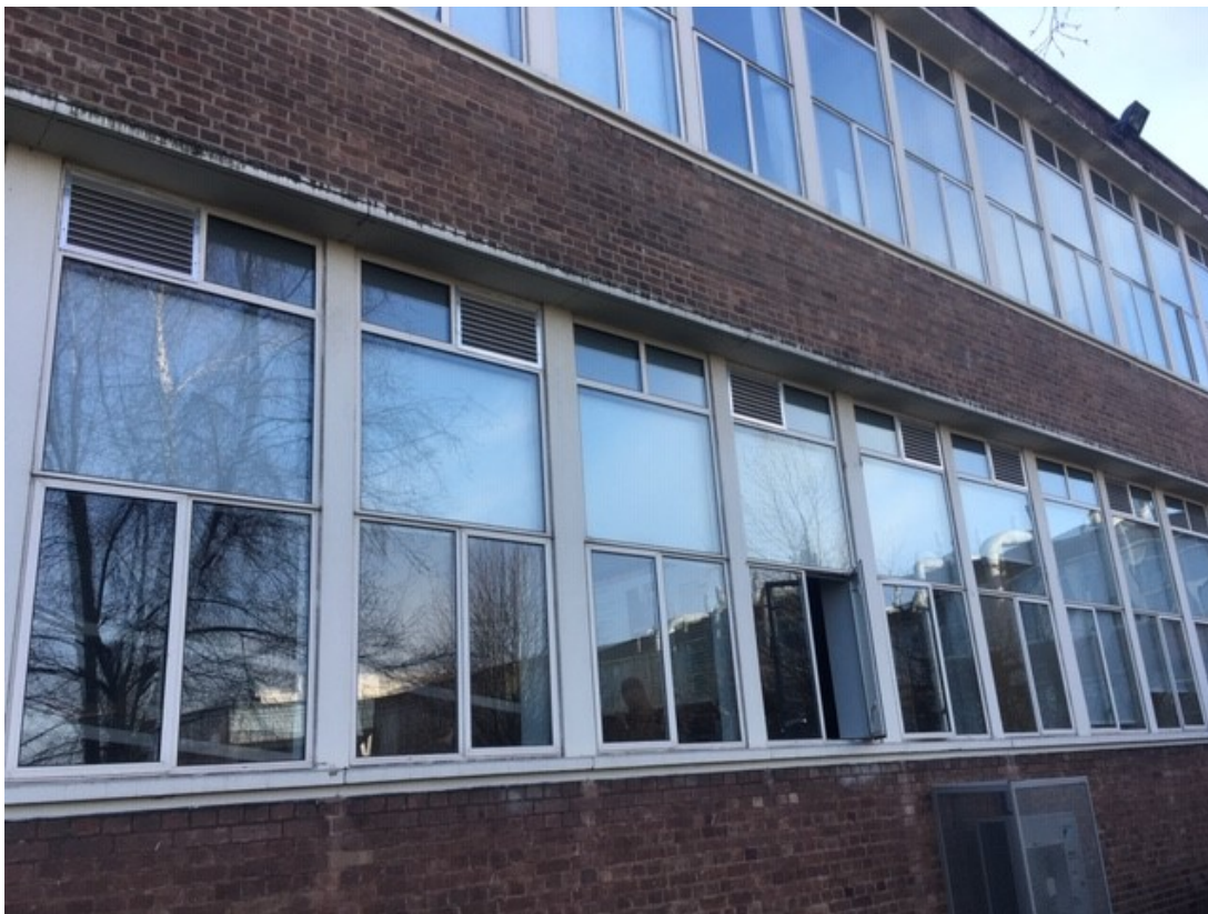
Image EDP 8: View of the louvered vents as employed on a different part of the building.
