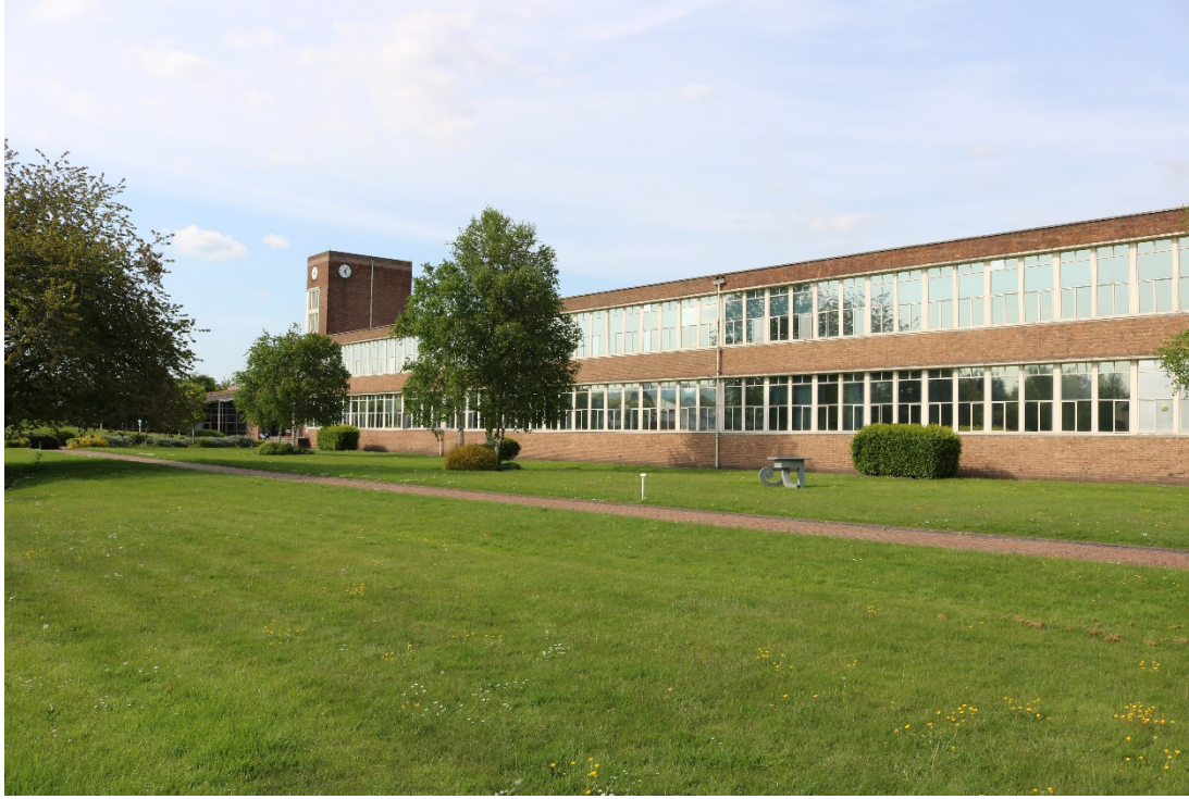
Image EDP 1: View of Block B from Mold Road.
