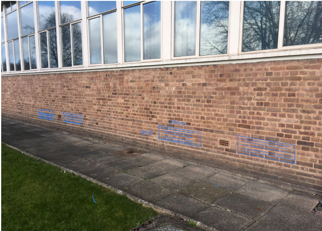
Image EDP 11: Sketched photograph illustrating the position of proposed vents in brickwork.
