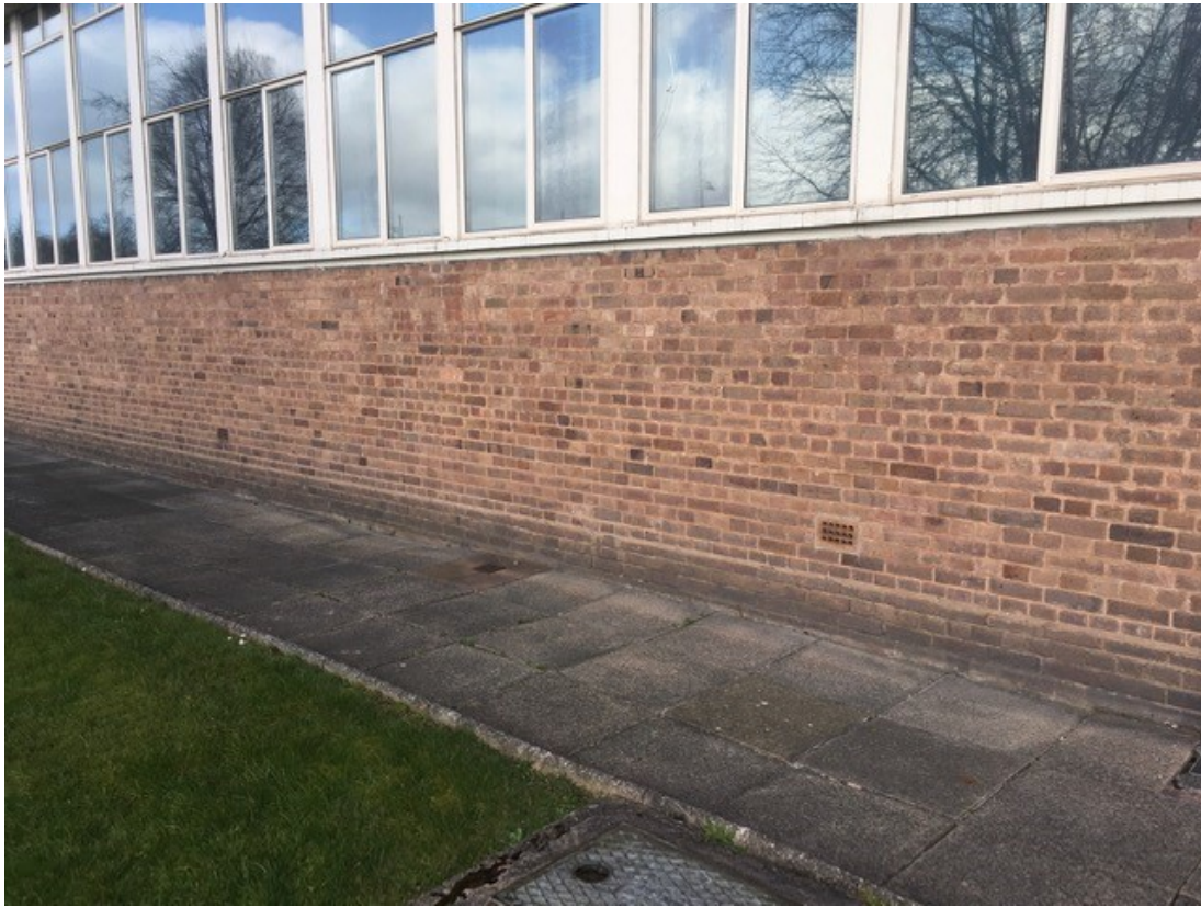
Image EDP 2: Detail of the lower brick band on the Mold Road elevation.
