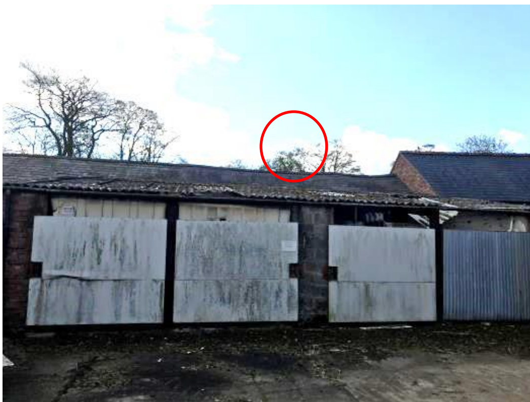
Plate 7 – Northern elevation of the western wing with asbestos-roofed lean to
