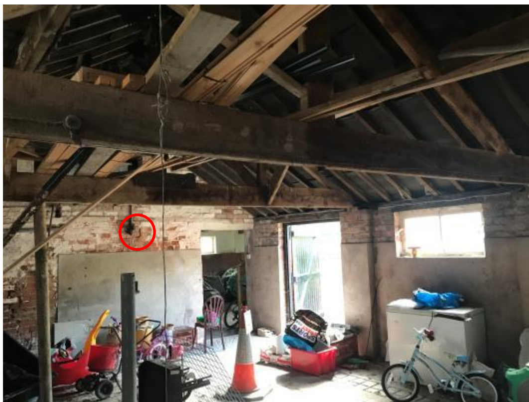
Plate 10 – Internal character of the western wing with bitumen 1F underfelt and internal crevices
