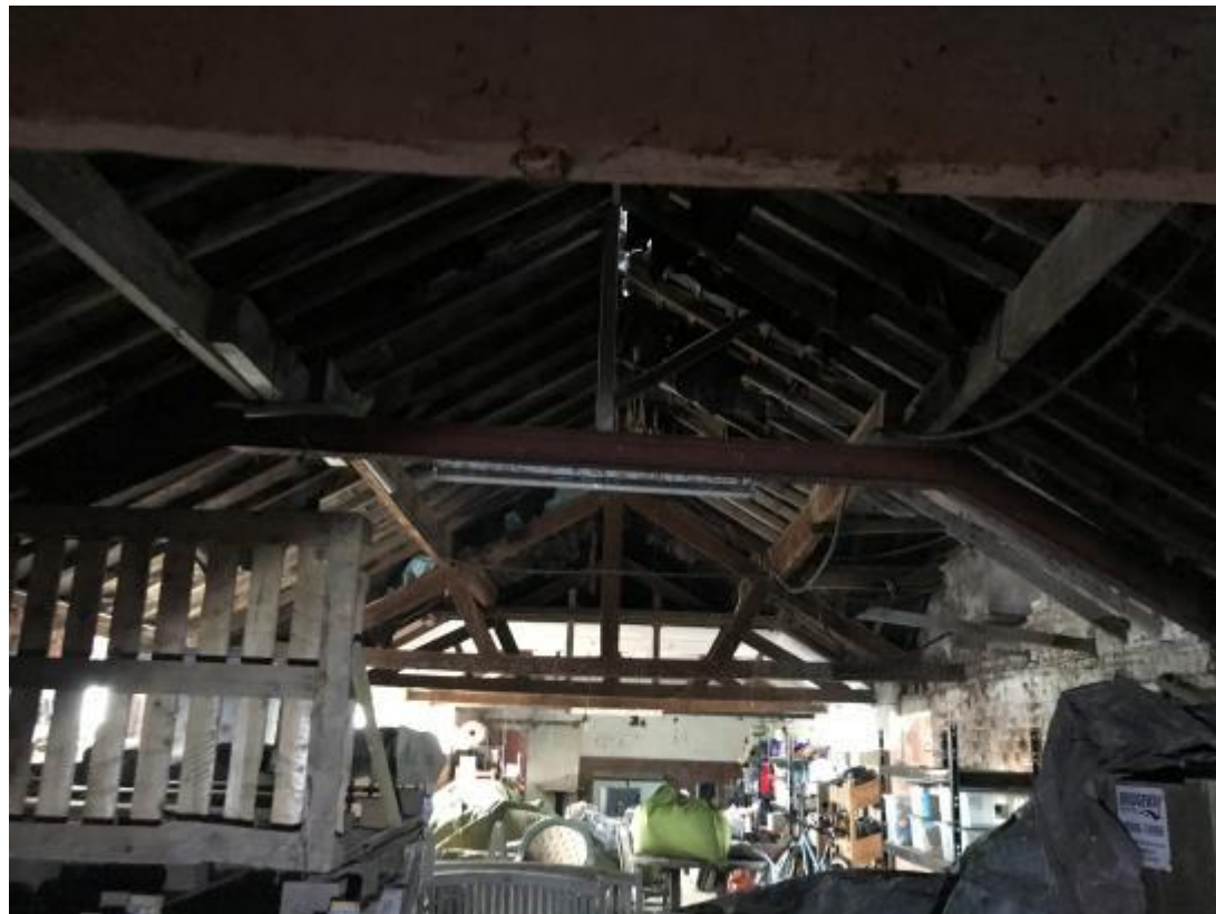
Plate 18 – Internal character of the eastern wing
