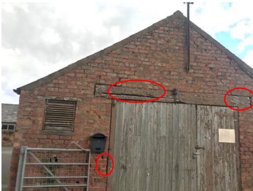
Plate 4 – Southern elevation of the eastern wing with abundant PRFs around the wooden barn door
