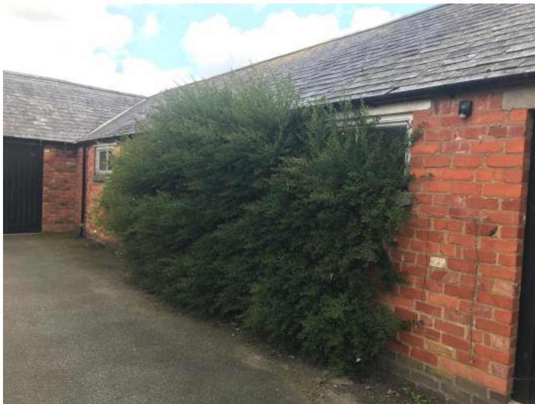
Plate 3 – Western elevation of the -eastern wing of the barn, with bushy vegetation that may be used by nesting birds
