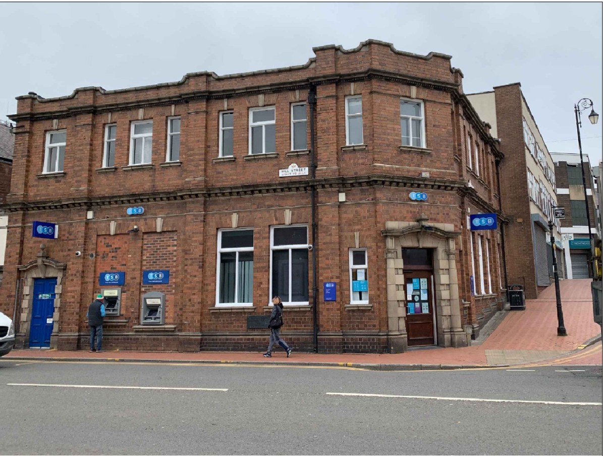
STREET SCENE TO TSB BRANCH
