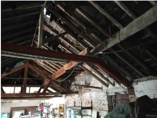
Photo 13 – General view of roof over barn.
