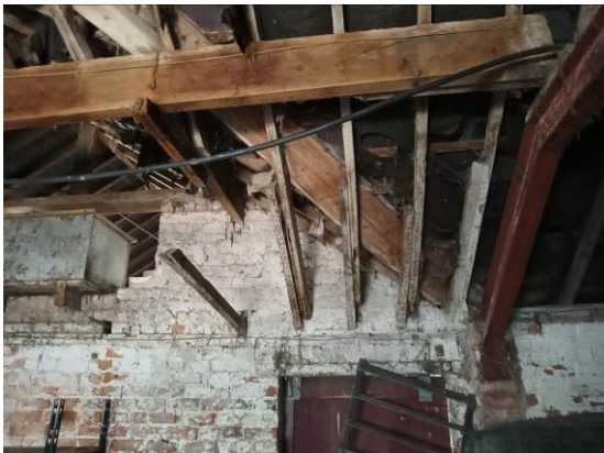
Photo 14 – General view of roof at intersection.
