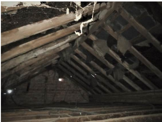
Photo 8 – General view of roof over store.
