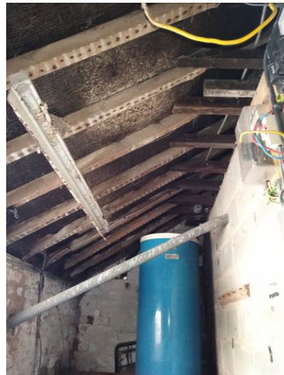
Photo 11 – General view of roof over WC.
