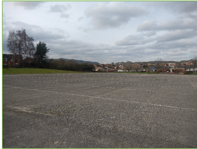
Plate 7: Example of hardstanding on site.
