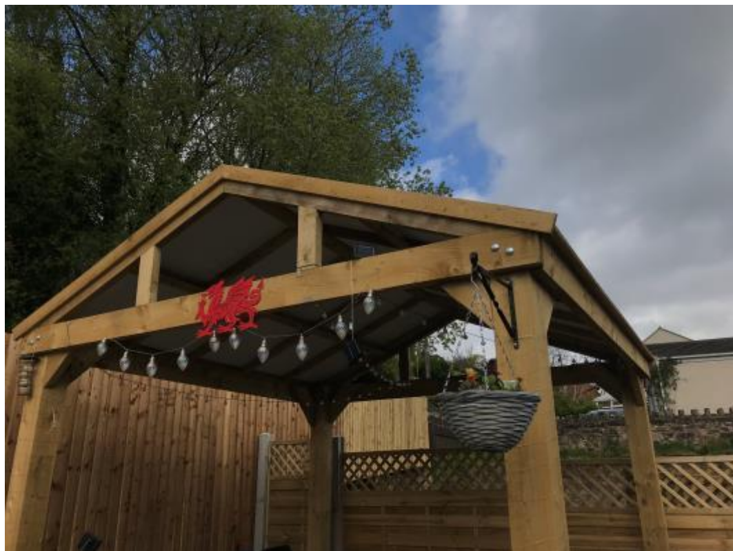
Plate 9 – Area of decking with a wooden shelter to the rear of the dwelling
