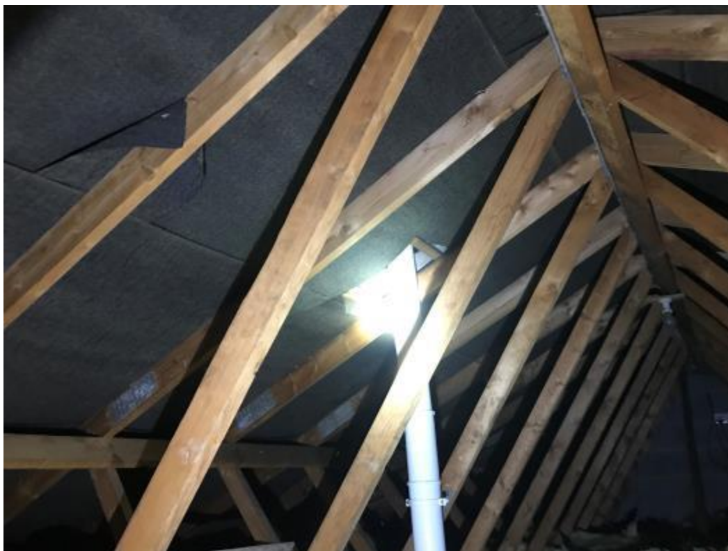
Plate 7 – Bitumen 1F underfelt roof lining
