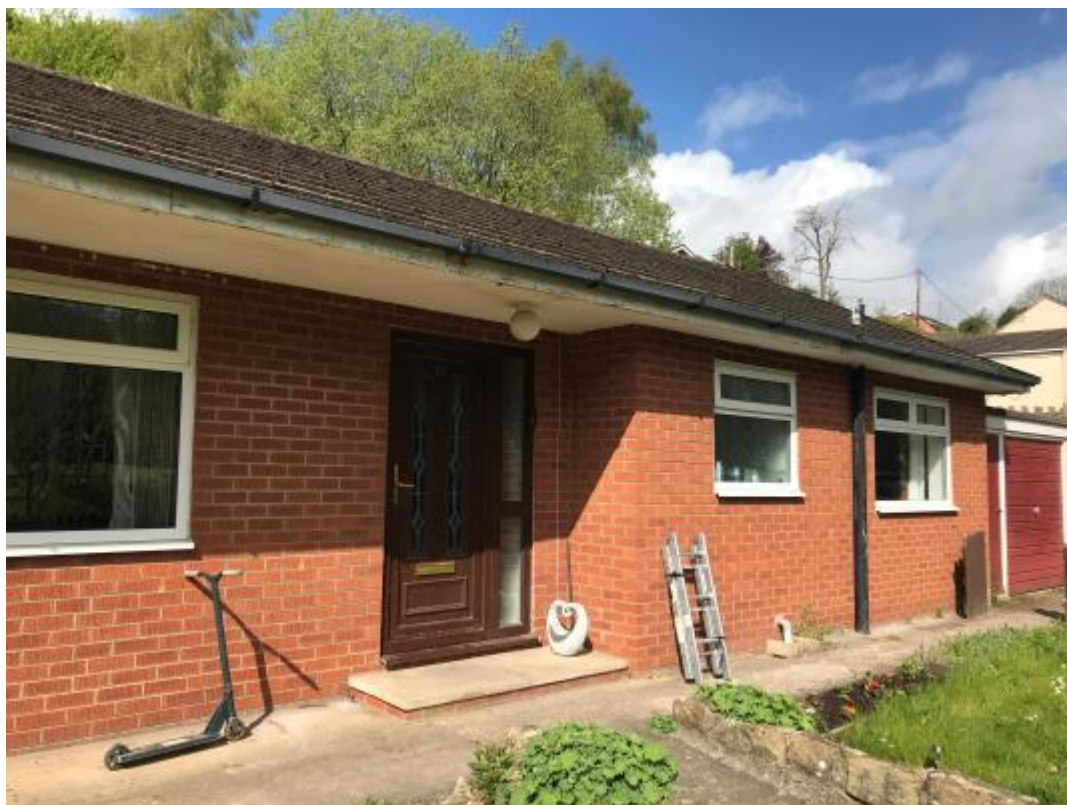
Plate 1 – Front elevation of the dwelling 33 Moss Hill
