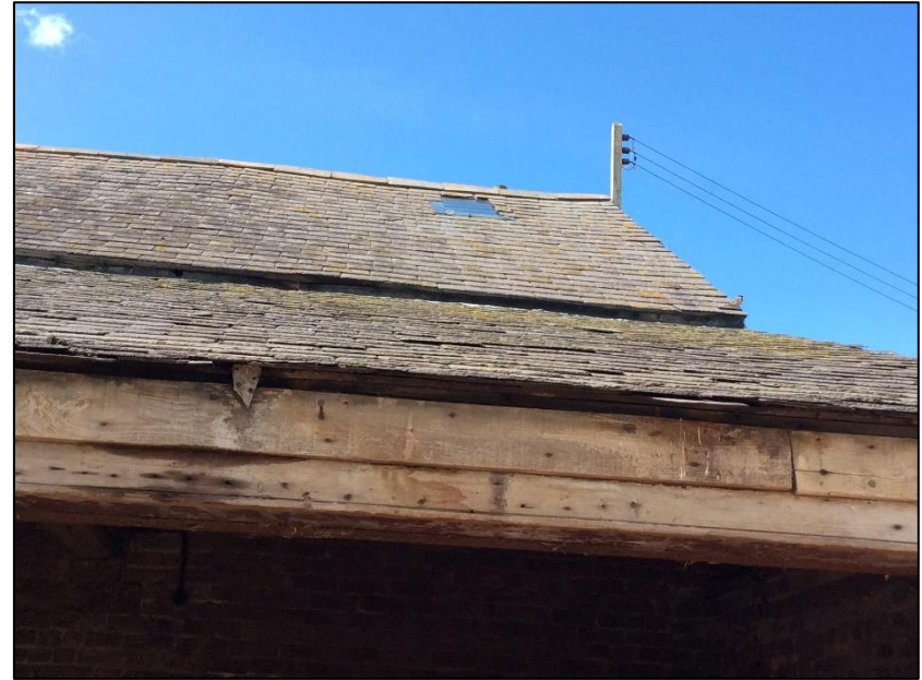
Raised tiles on the eastern elevation.
