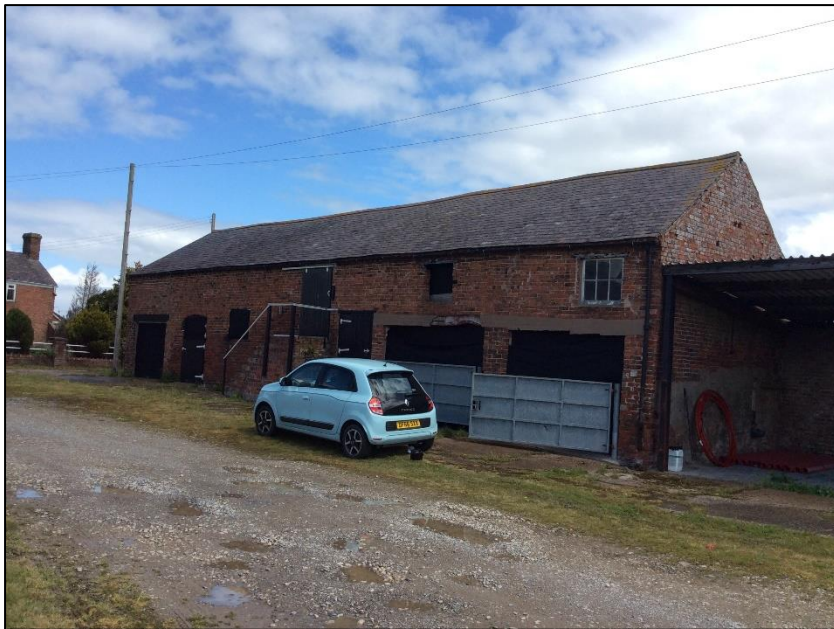
Western and southern elevations.
