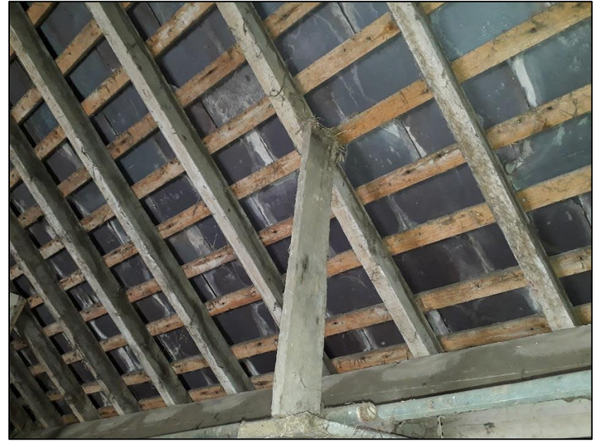
Tight-fitting roof tiles.
