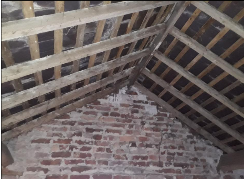
Northern gable end.
