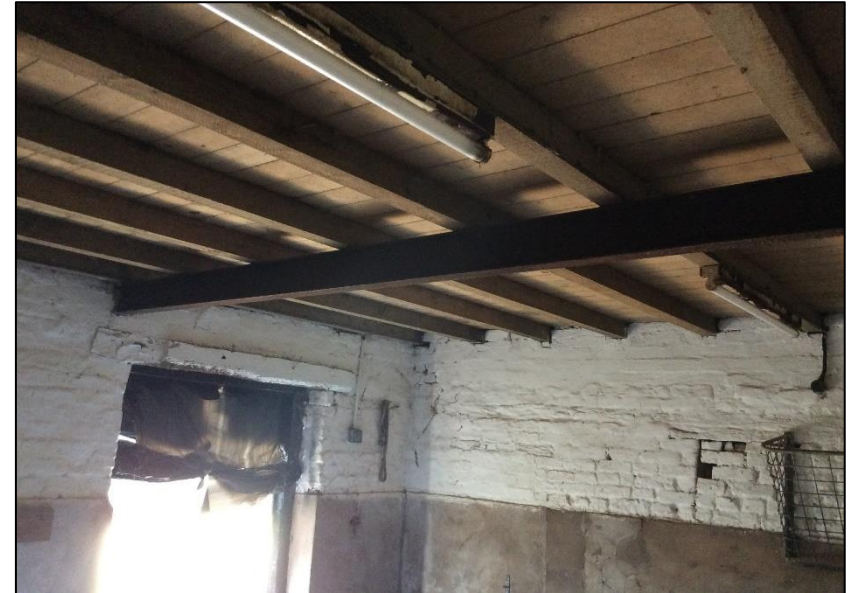
Ground floor of the barn.
