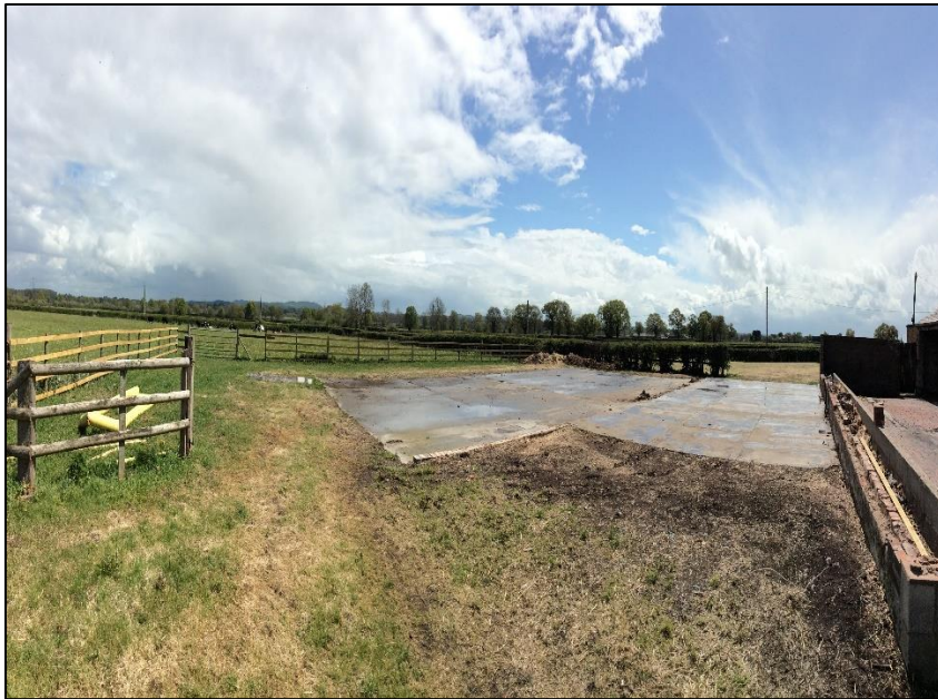
Eastern section of the site.
