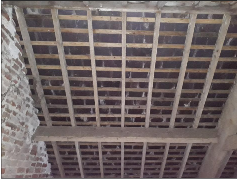
Tight-fitting roof tiles.
