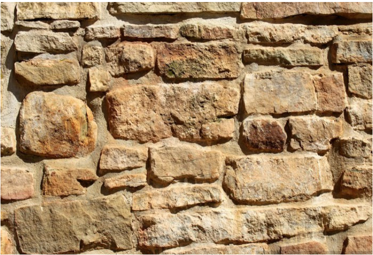
Low level stone wall
