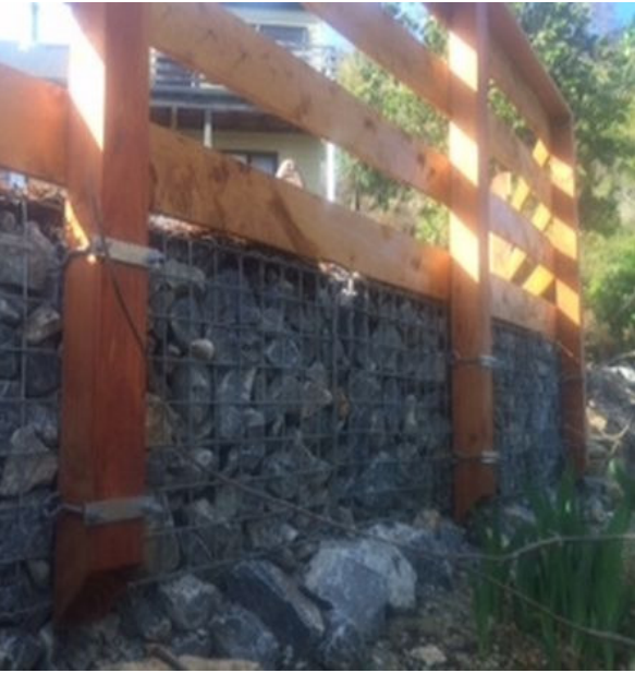
Post and rail fence above gabion baskets.
