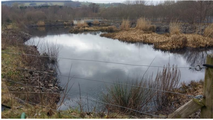
Photo 8. Lagoon 3 – Settling and water treatment facility for operational facility
