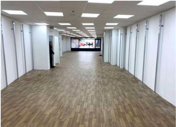
The existing retail unit at ground floor
