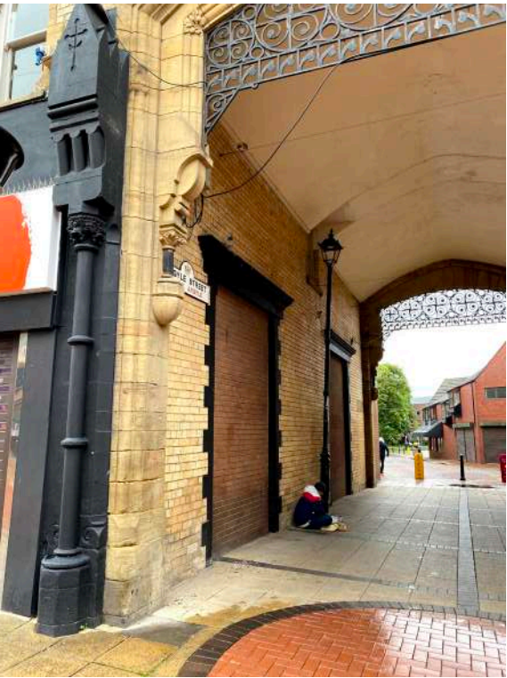
Archway looking towards Argyle Street
