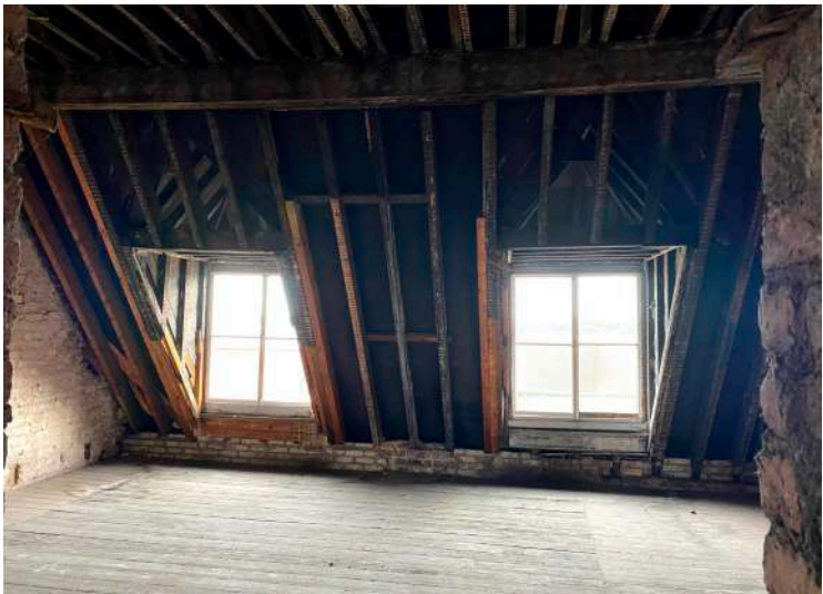
Vacant top floor - stripped back to brickwork
