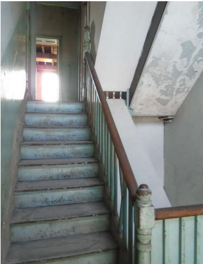
Existing staircase to be reused and restored as part of the works
