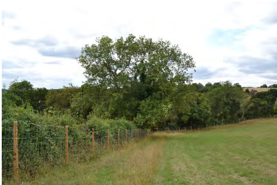
Figure 1 – Example of c.2m high deer fencing.
