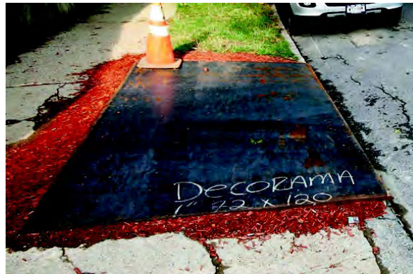
Figure 2: Steel plates atop a layer of woodchip and a breathable geotextile membrane.
