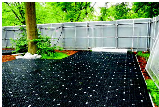
Figure 3: ArborRaft system in use outside a CEZ.
