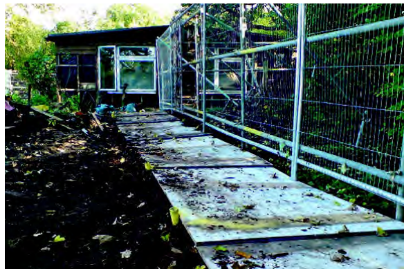
Figure 1: Plywood boards atop a layer of woodchip and a breathable geotextile membrane.
