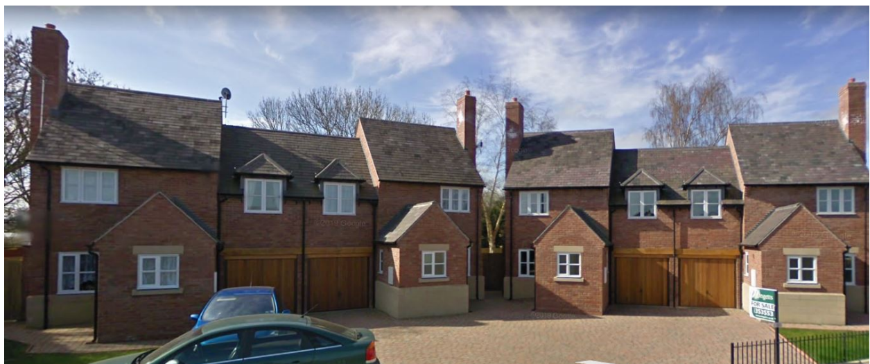
Fig.6 Recently completed new housing.
