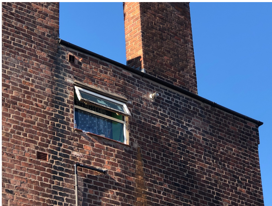
FIGURE 1: Image of the rear elevation of existing flue.
