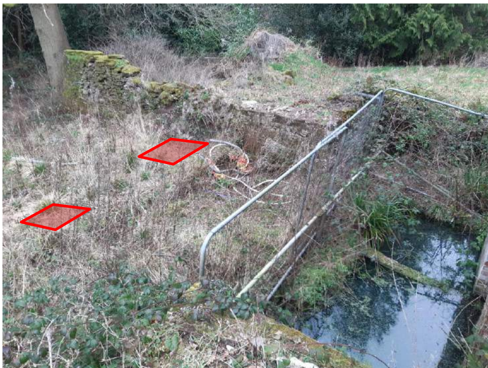
Figure 1 Approximate location of concrete pads
