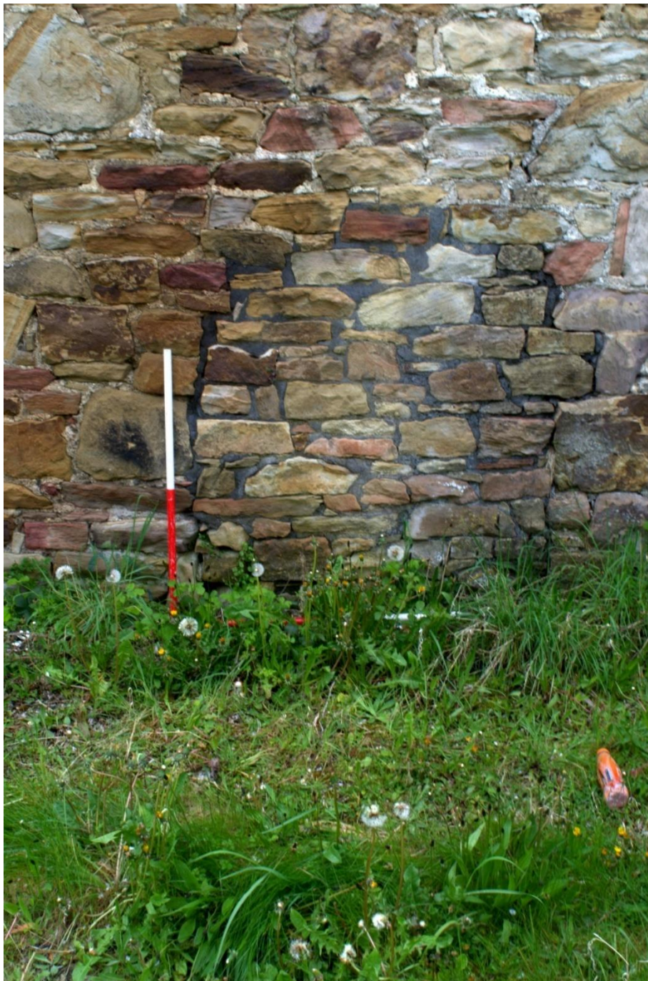
Figure 40 West elevation West Range blocked former opening
