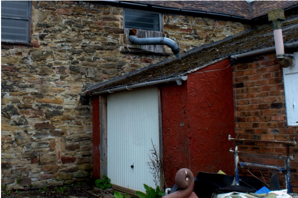
Figure 23 East elevation of West range with lean-to outshot
