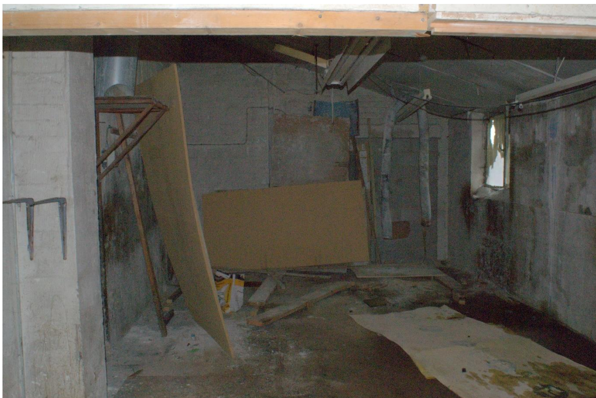
Figure 46 Lean-to West room interior looking East Middle window on Right
