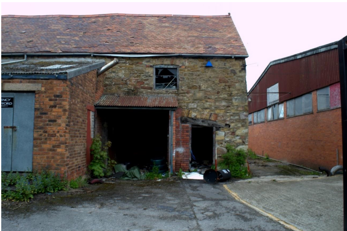
Figure 24 North range East end of South elevation
