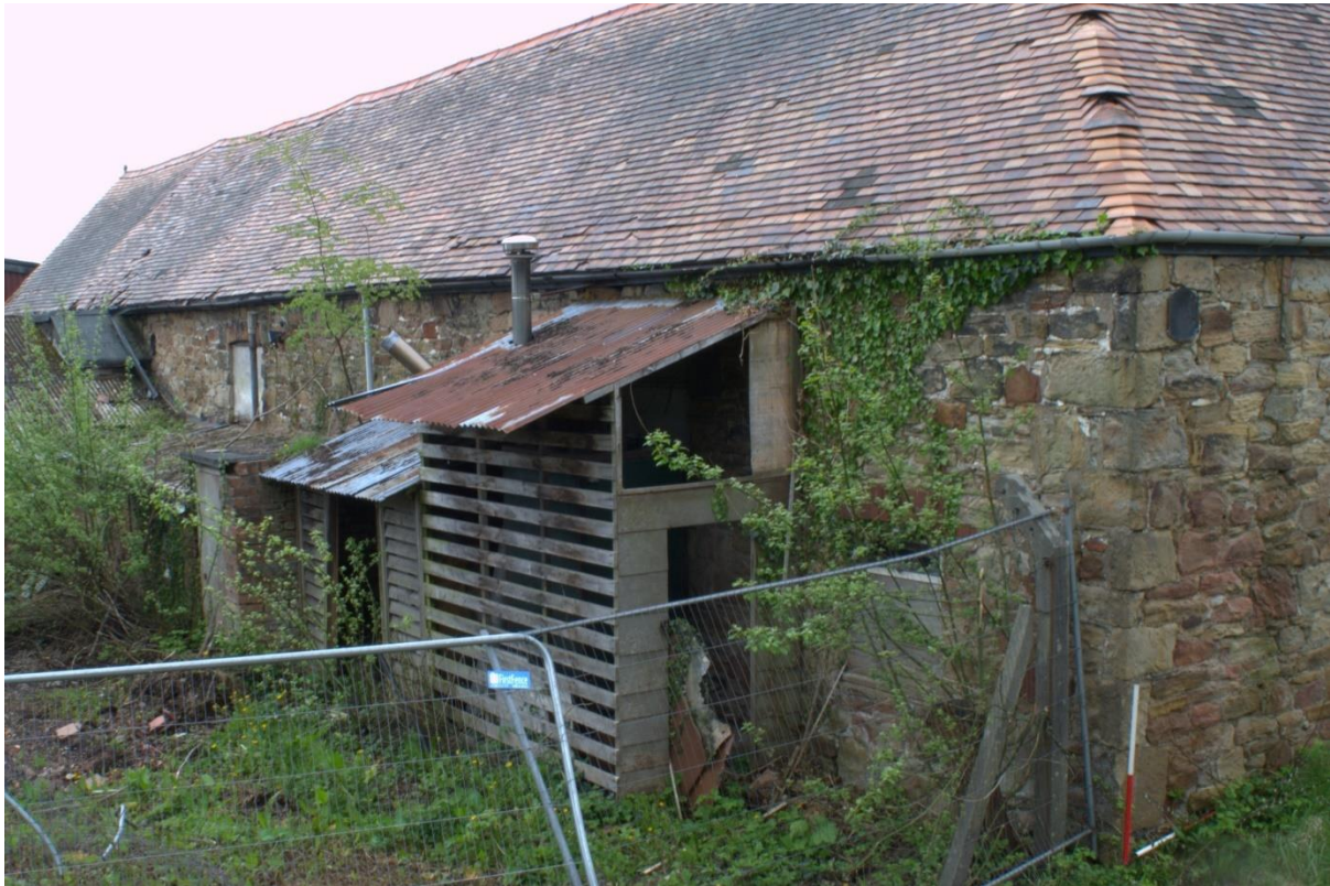
Figure 15 North range, north elevation, later lean to structures.
