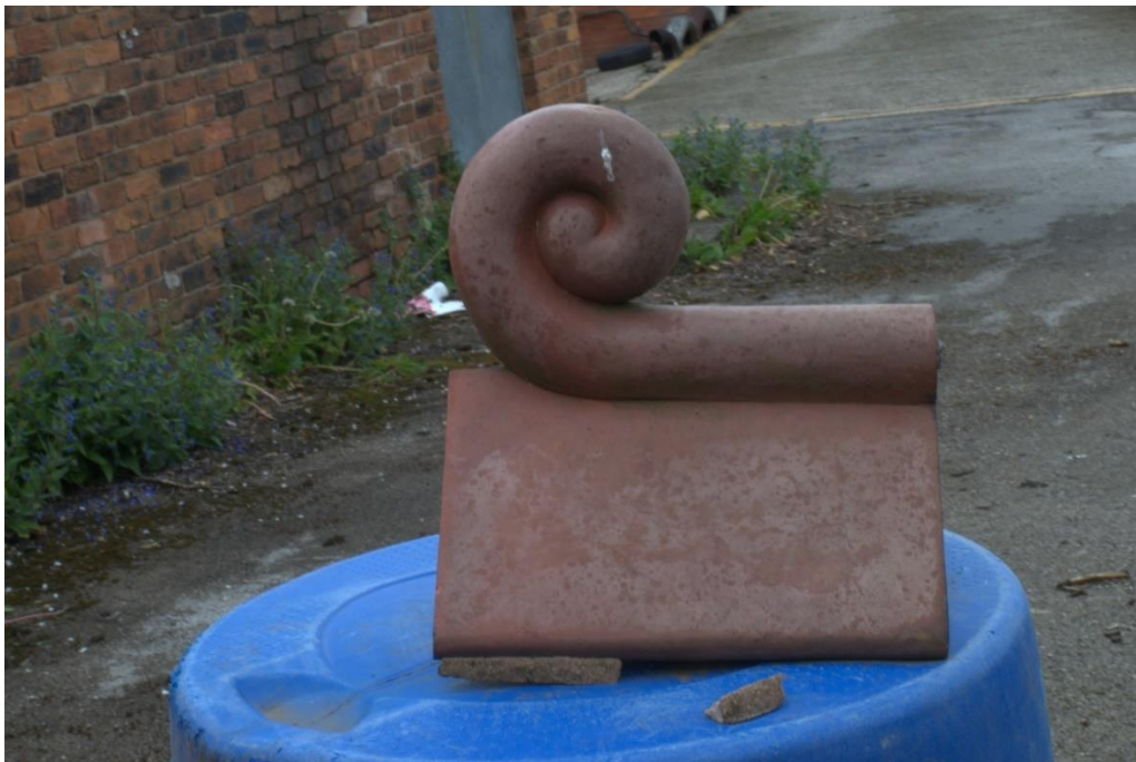
Figure 13 Ridge finial tile side view
