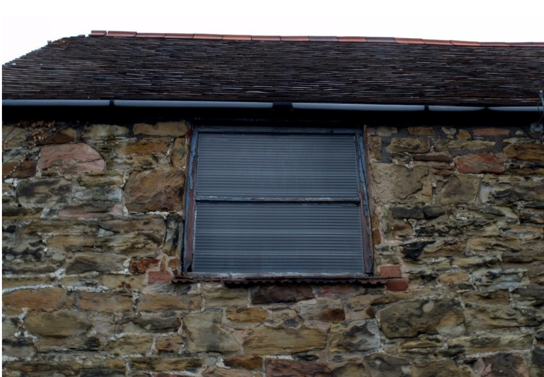
Figure 34 West Range, upper floor's window with metal sheet blocking
