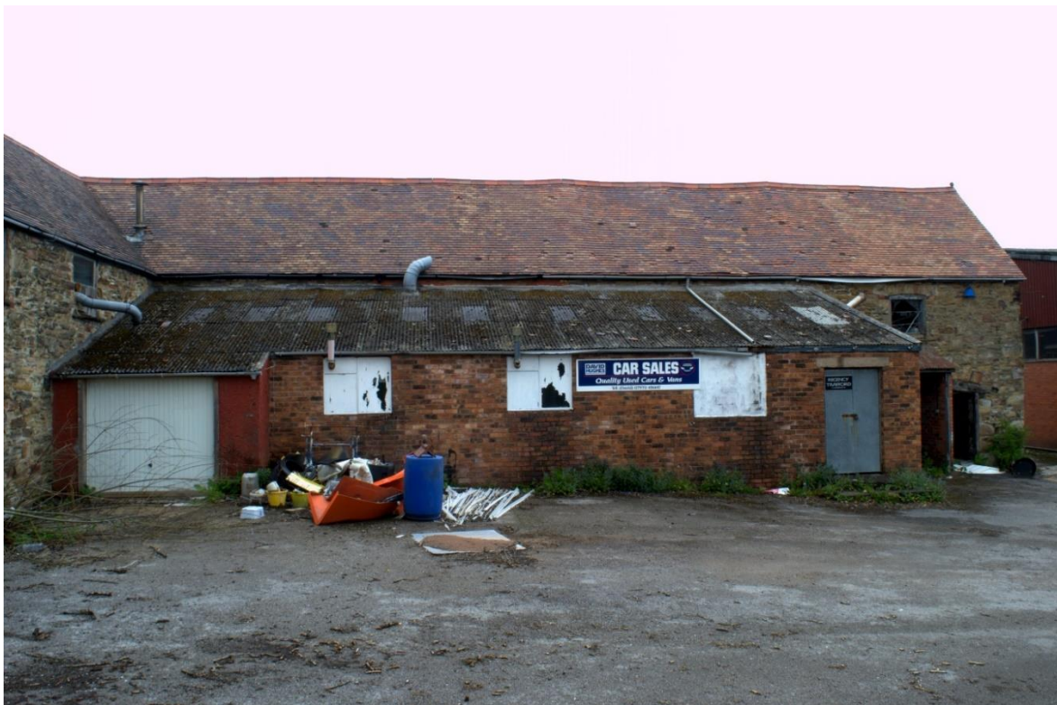
Figure 22 Lean-to on South elevation of North Range
