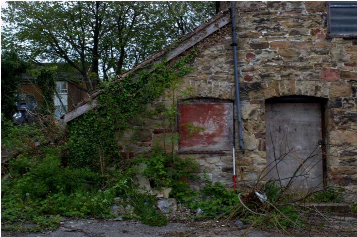
Figure 27 Upper floor window at E end of South elevation of North Range
