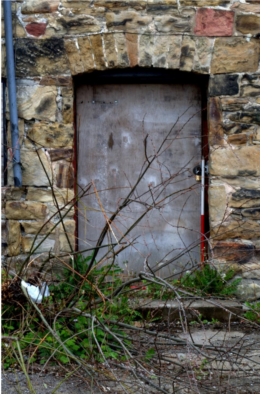
Figure 32 Detail of door at South end East elevation of West Range
