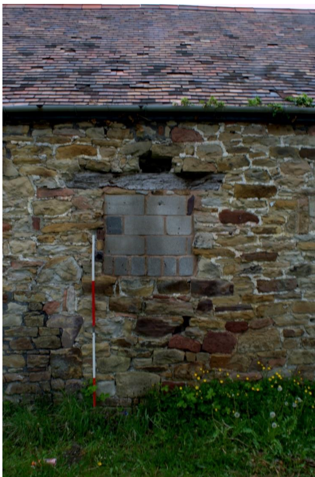
Figure 41 West elevation West Range blocked pitching door
