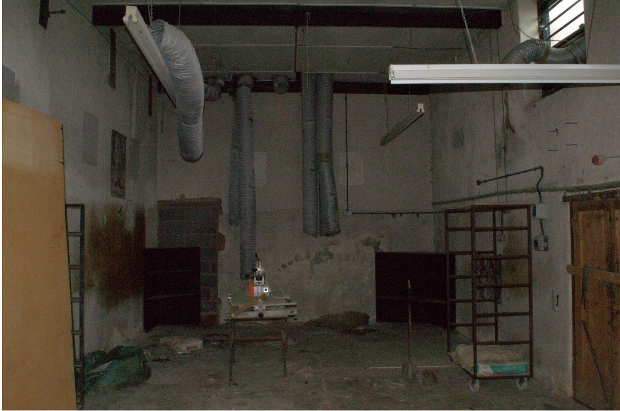
Figure 45 West range interior from Southern end
