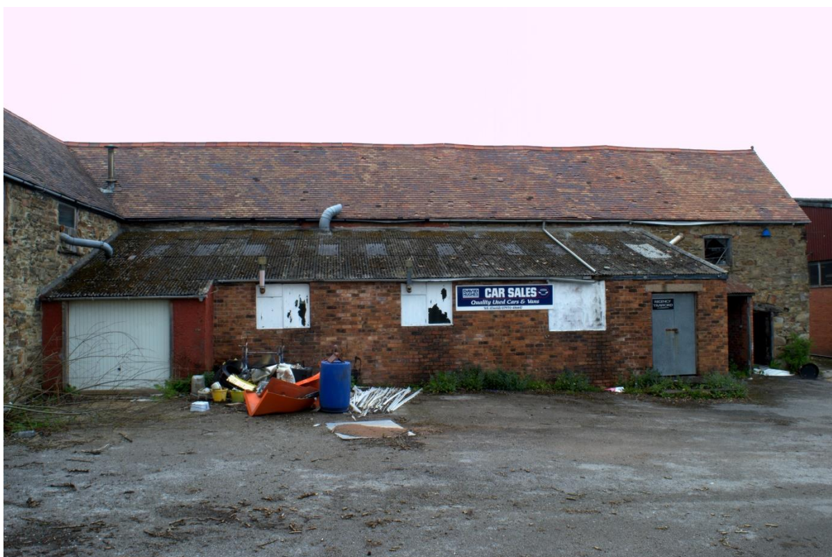
Figure 11 North range South elevation with added brick lean-to
