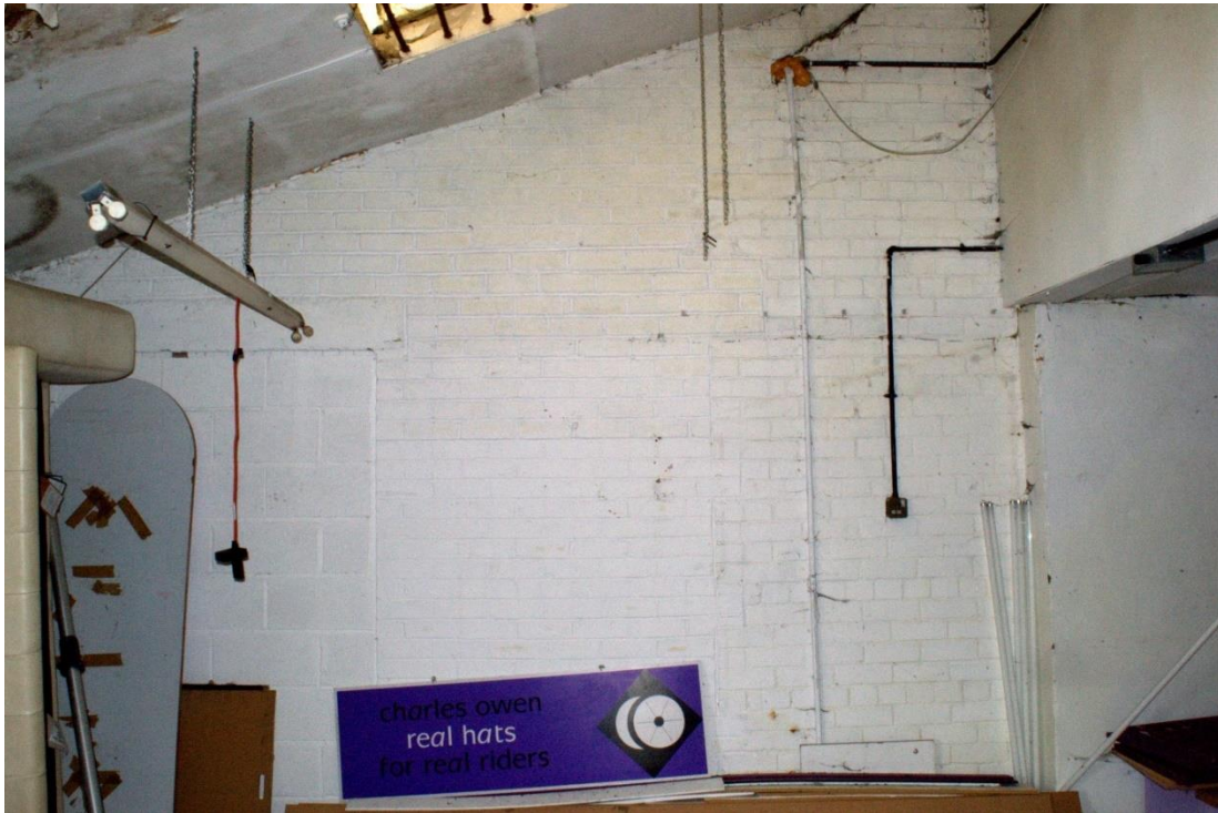
Figure 48 North range lean-to East room West elevation partition wall
