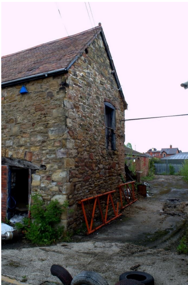
Figure 19 East gable of North Range from SE
