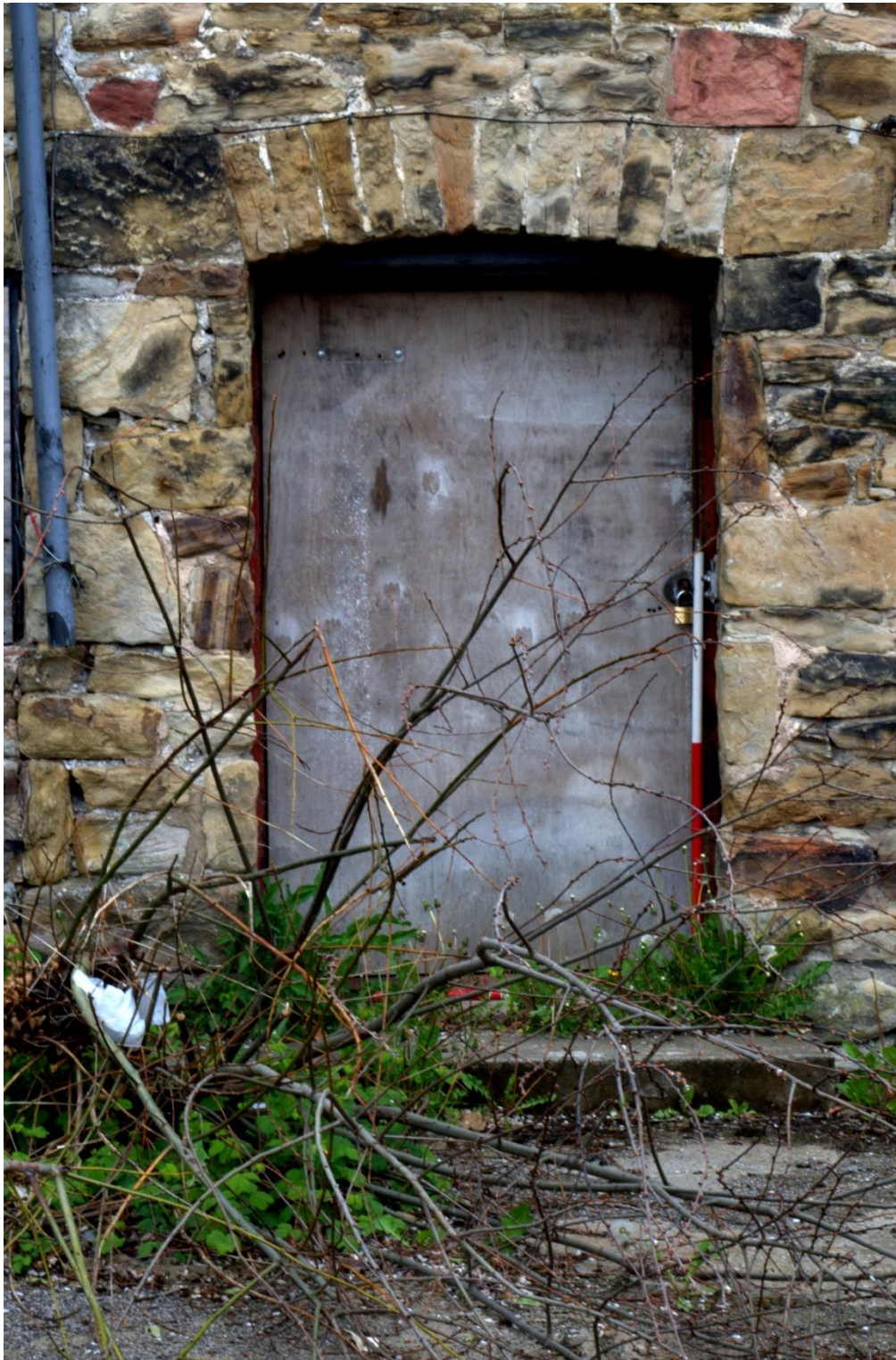
Figure 33 E elevation of barn blocked ventilator
