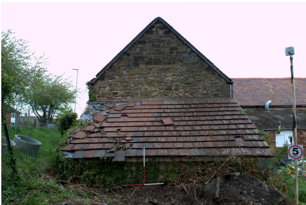
Figure 10 West range South gable and South lean-to
