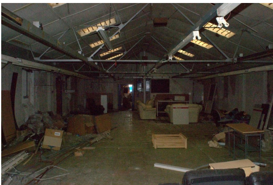
Figure 44 Brick shed Interior view to South
