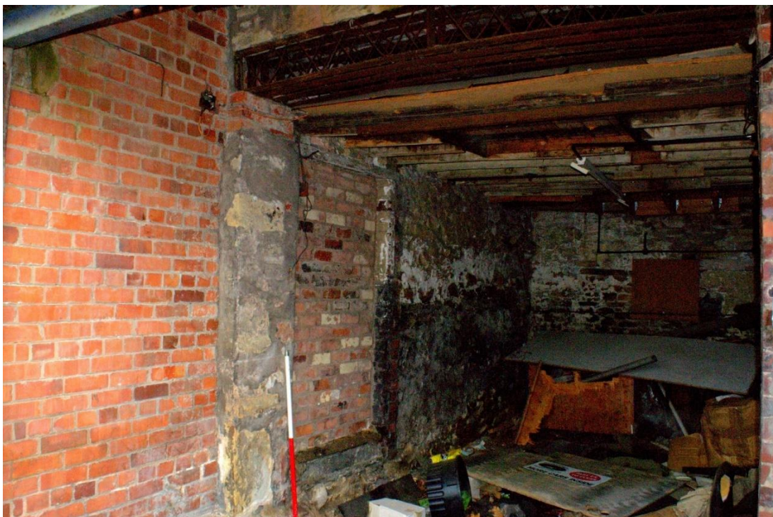
Figure 49 North Range room behind large opening at Eastern end West elevation with blocked doorway
