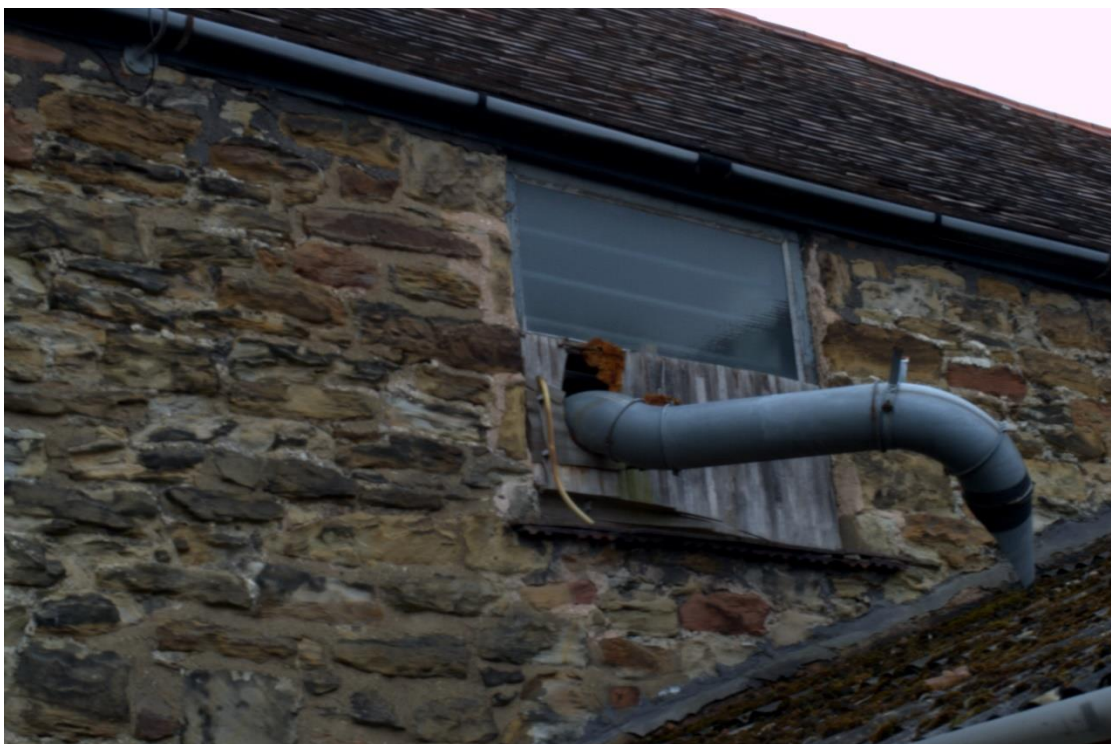
Figure 35 West Range, upper floor n window with ventilator pipe
