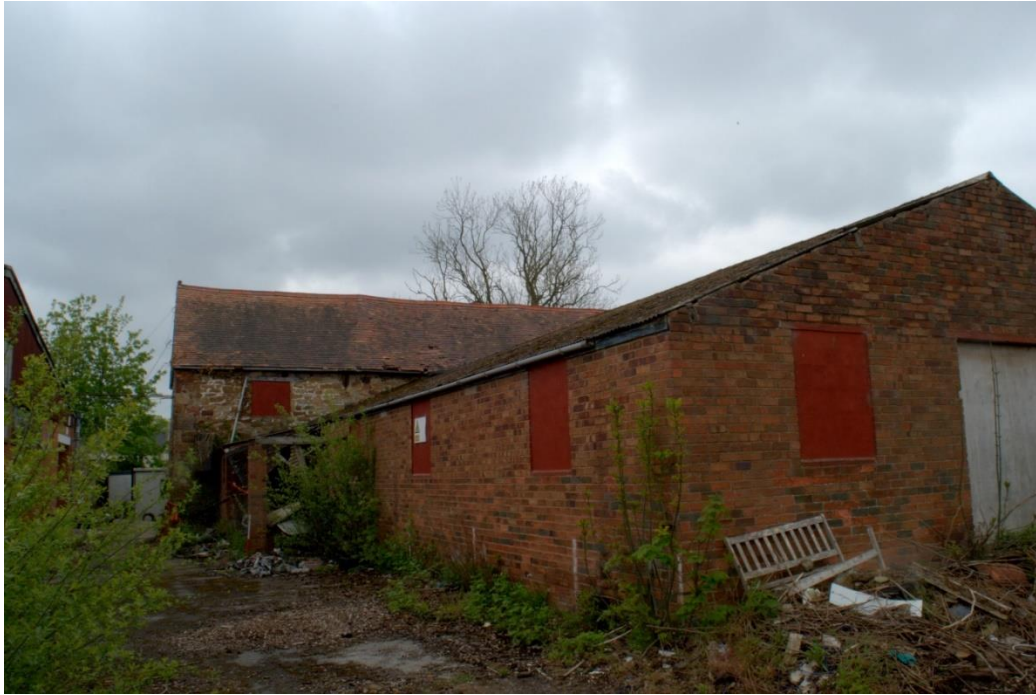
Figure 16 Brick shed addition to E end North elevation of North range from NE
