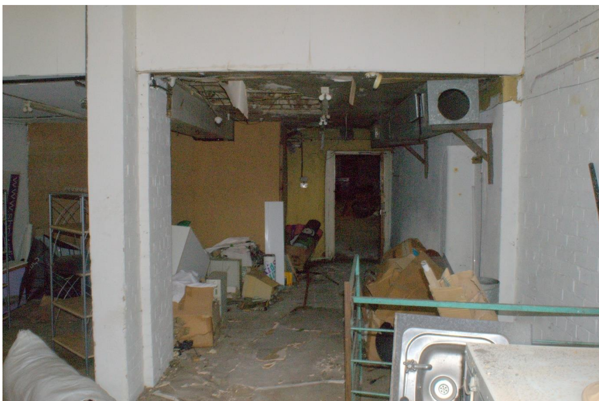
Figure 47 North range barn interior from lean-to
