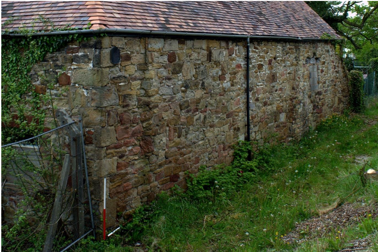
Figure 36 Western elevation of West Range from NW
