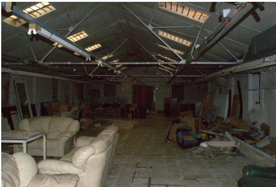
Figure 43 Brick shed Interior view to North
