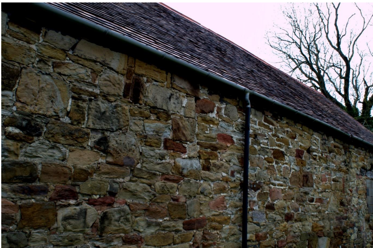
Figure 39 West elevation West Range Vertical straight joint
