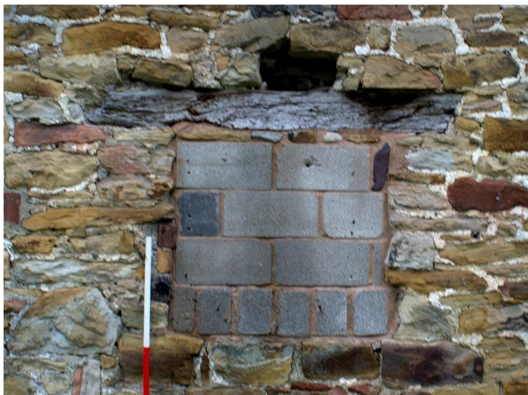
Figure 42 West elevation West Range blocked opening detail
