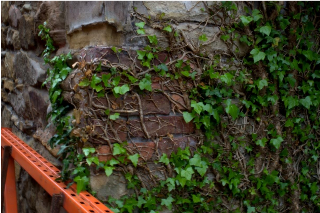
Figure 21 Brick patch replacing stone quoin NE corner of North range
