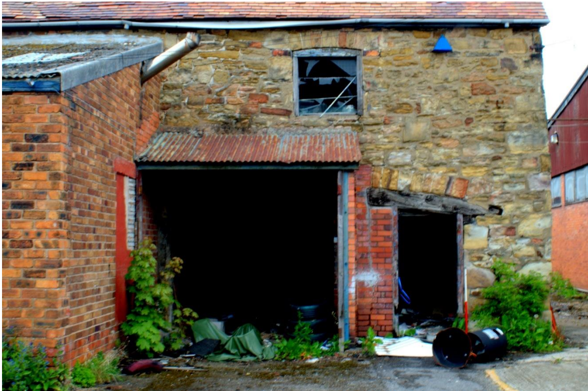
Figure 26 Altered original and later inserted openings at Western end, South elevation North Range
