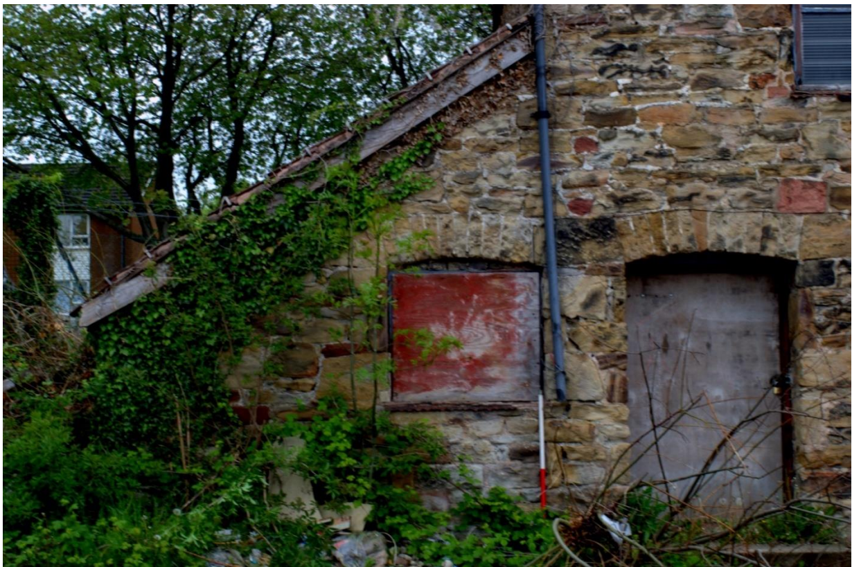
Figure 28 East elevation of lean to on South gable of West range
