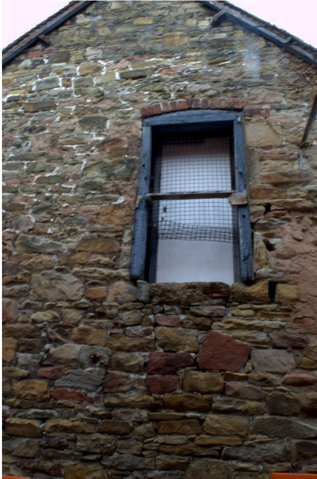
Figure 20 East gable window
