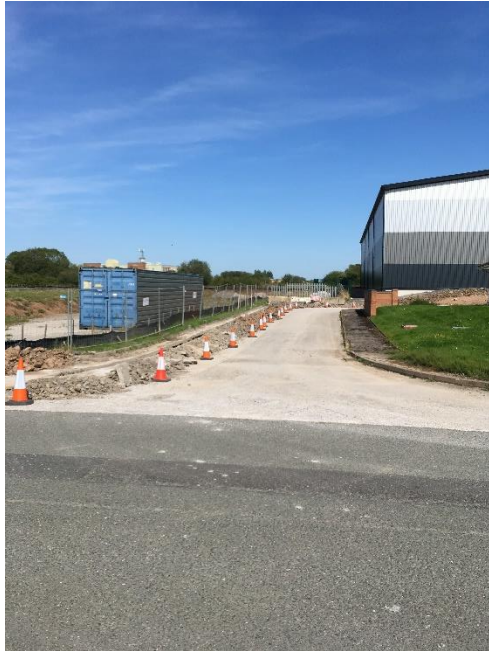
Photograph 1 – Site Access Road
