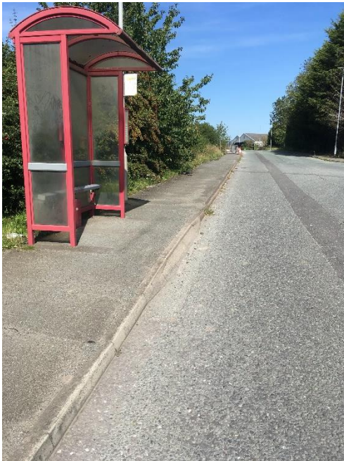
Photograph 3 – Bus Stop Infrastructure Bridge Lane North
