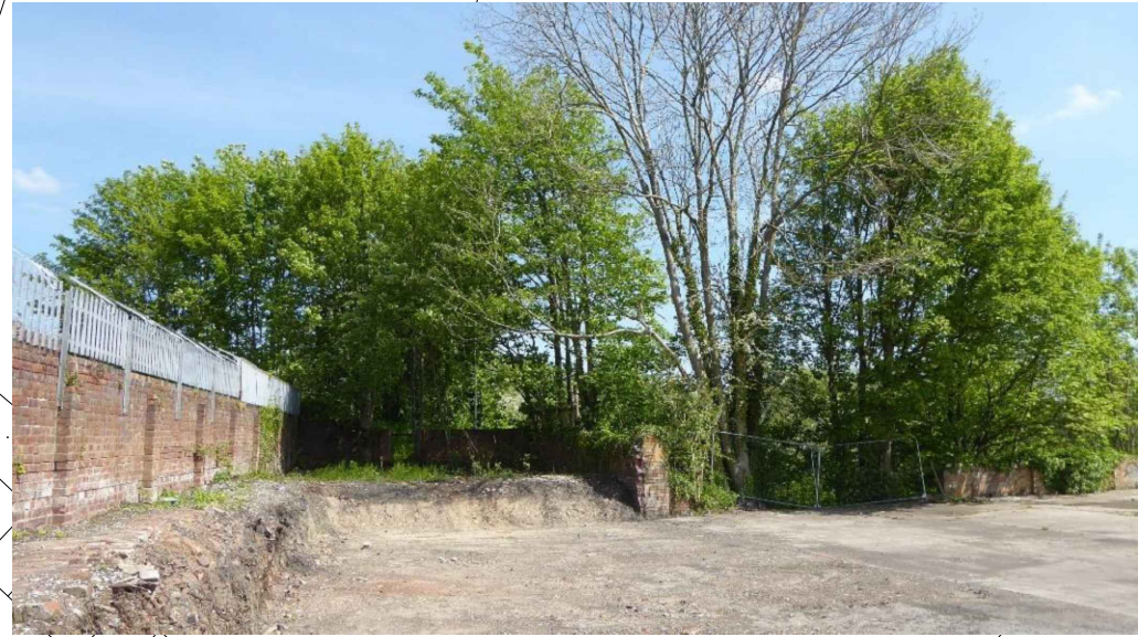
Photo looking towards north of site
