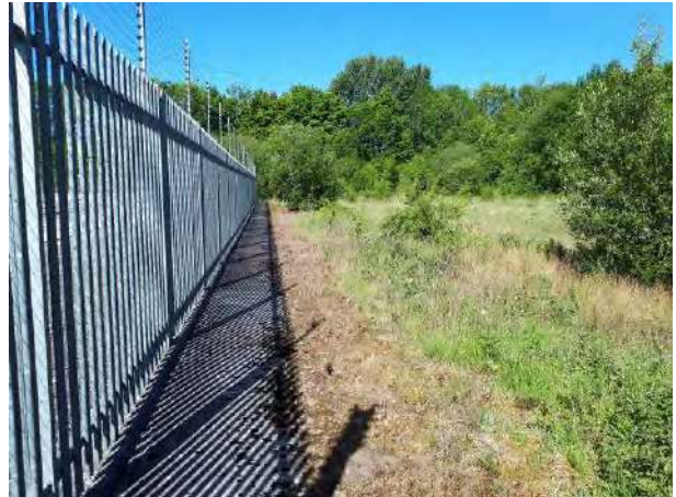
Main site's southern boundary formed by palisade fence of substation
