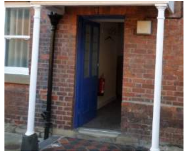
Cast Iron Pilasters
