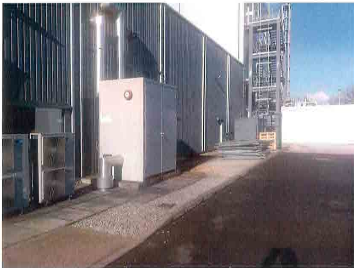
Photograph 2: Existing Building 55, facing south.
