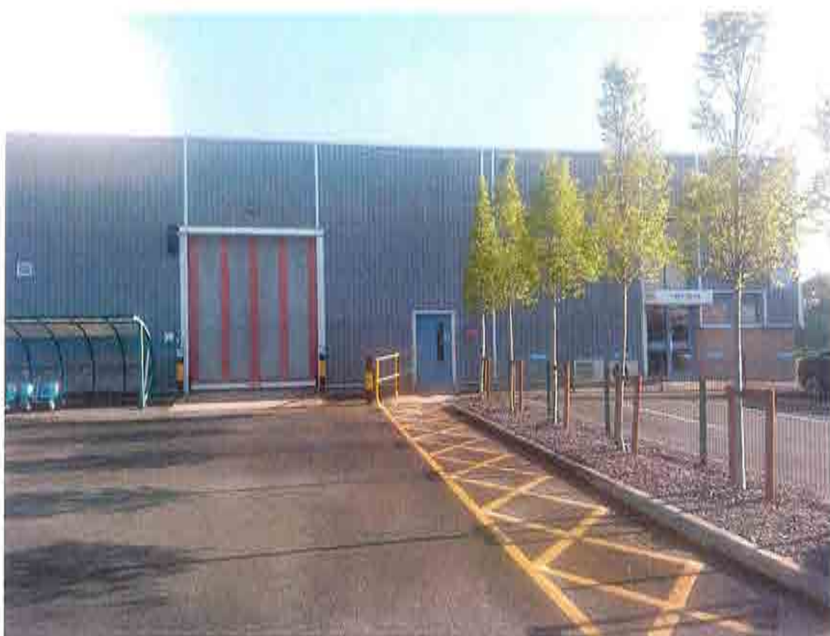
Photograph 1: Existing Building 55, facing north.
