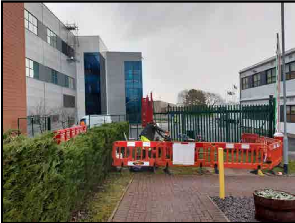
Photograph 1. Looking south at borehole location in grass.
