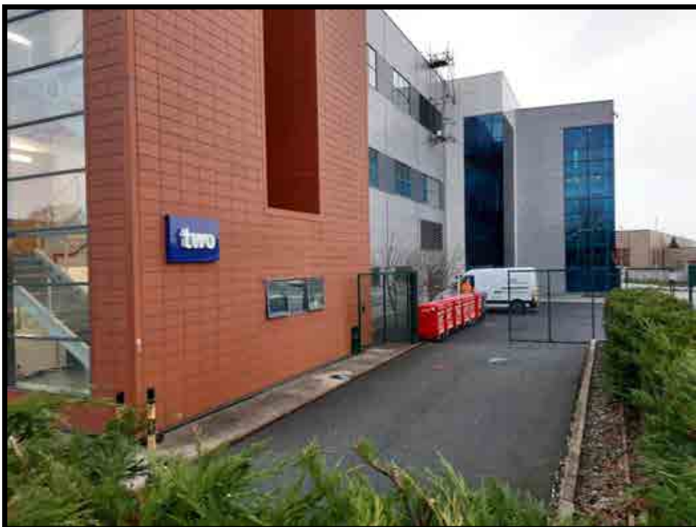
Photograph 2. Looking southeast at existing building Two.
